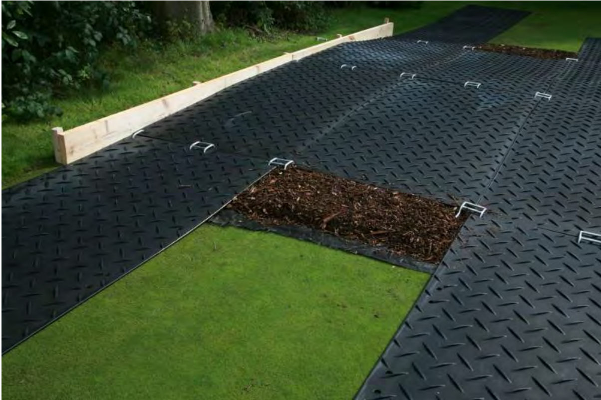
Figure 4: Ground protection example showing a combination of woodchip and ground protection mats used to provide increased load spreading and reduce soil compaction.
