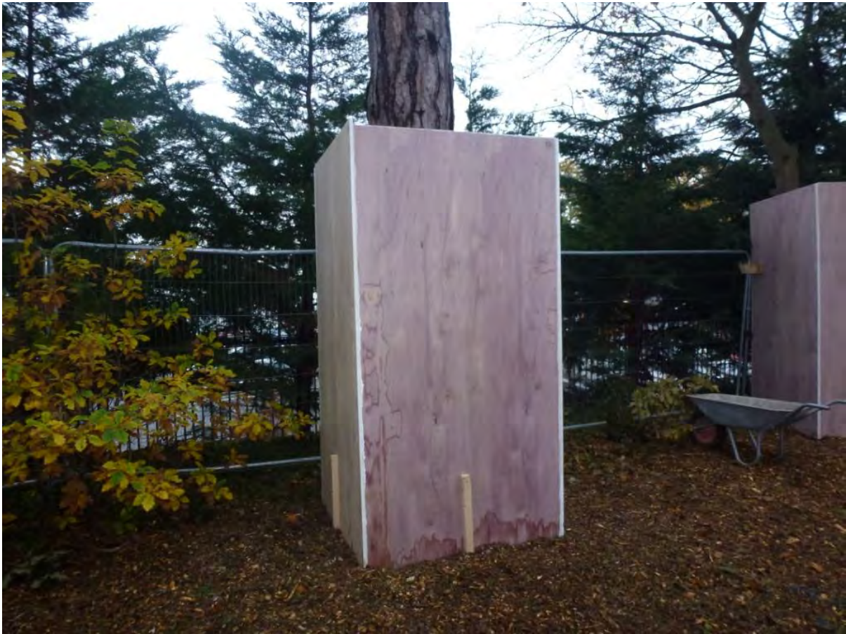
Figure 3: Example of plywood boxing supported by stakes, erected to protect the stem of trees within the working area.
