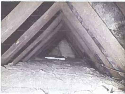
1. The original roof space within the main house.
