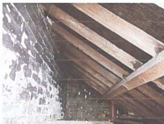
10. The roof space within the converted stable block.
