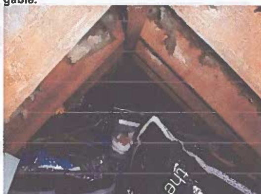
6. The newer roof space within the main house.
