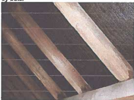
11. Bitumen roofing felt fully intact throughout.
