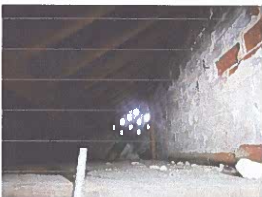
13. Ventilation bricks within the stone blockwork gable.
