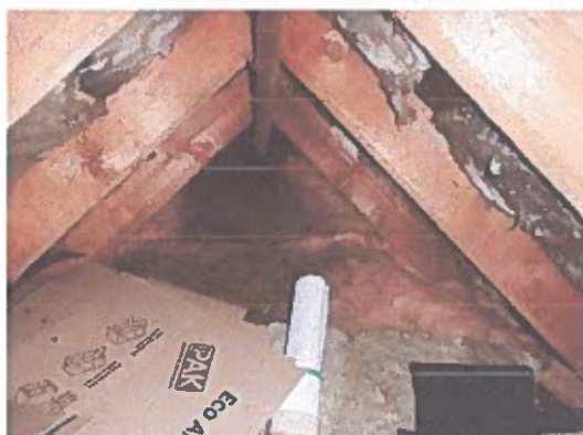
8. Eaves filled with fibreglass and void used for storage.
