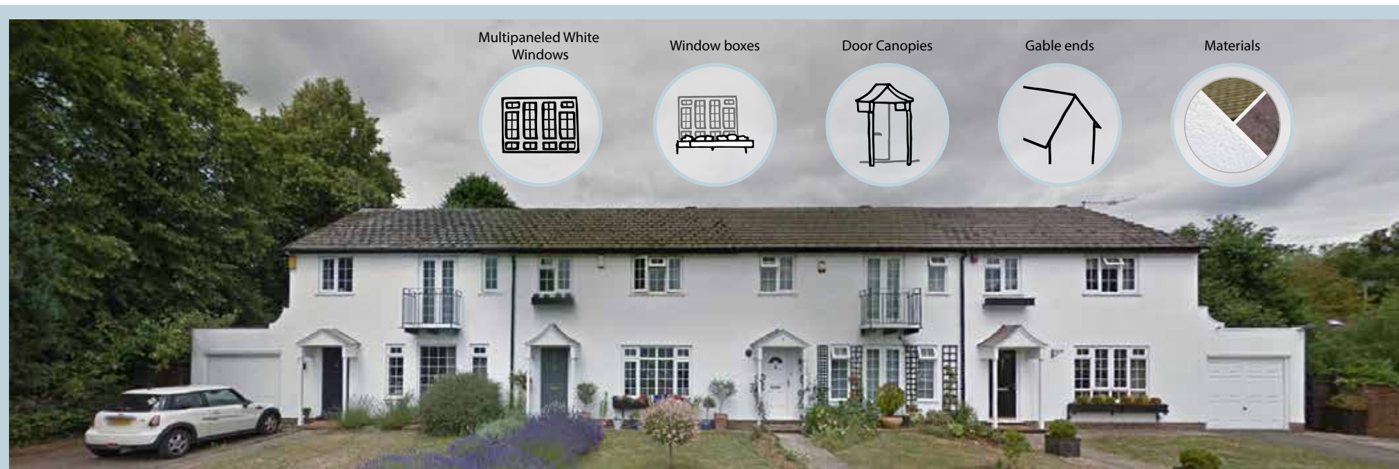
Figure 4: Example Facade for Wingrove Road and Hollins Walk Terraces (© Google Street View)
