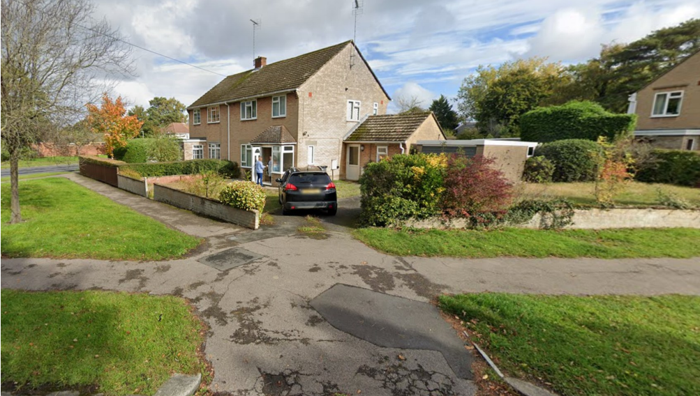
Fig.01 View of the site
