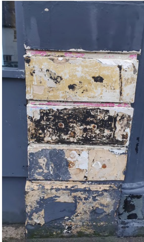
Poultice stripped pilaster
