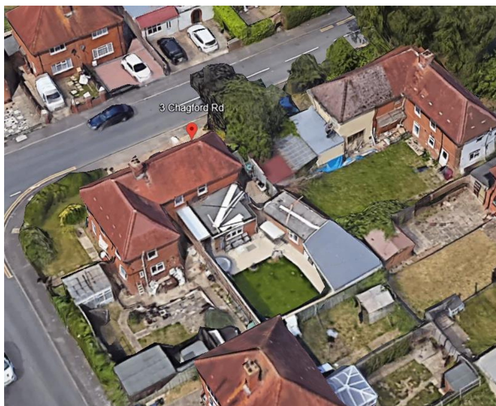
Aerial view of the rear of the property. Image taken from Google Earth on 2 May 2024.
