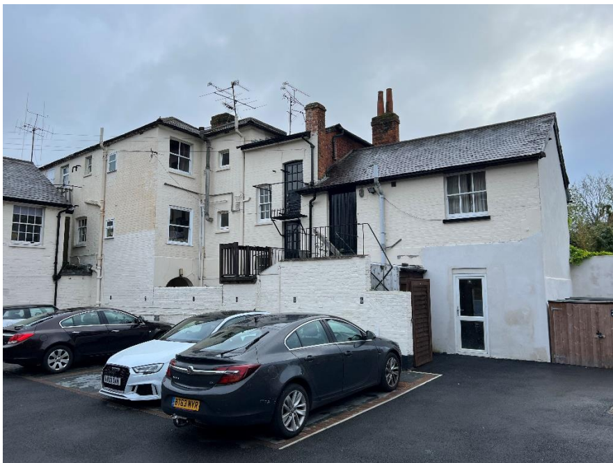
Side Elevation of 55 Baker Street
