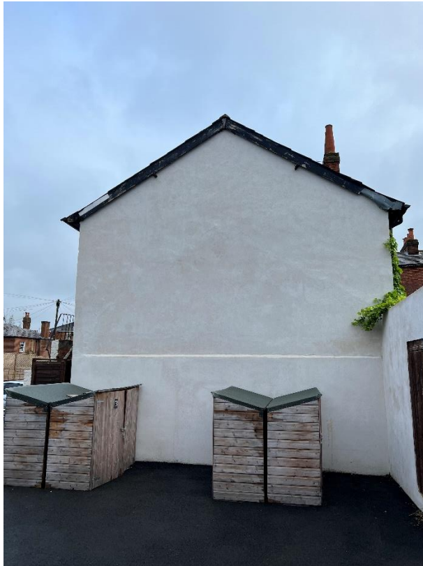
Rear Elevation of 55 Baker Street
