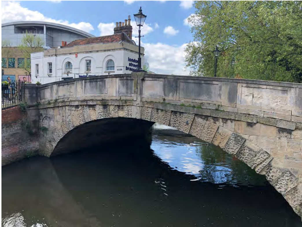
Figure 5.5: View of High Bridge from the waterside
