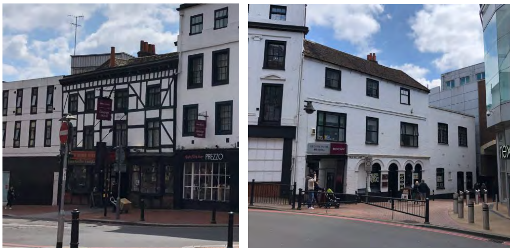
Figure 5.11: (2no) View of George Hotel, King Street and Building on south-east corner, Yield Hall Lane
