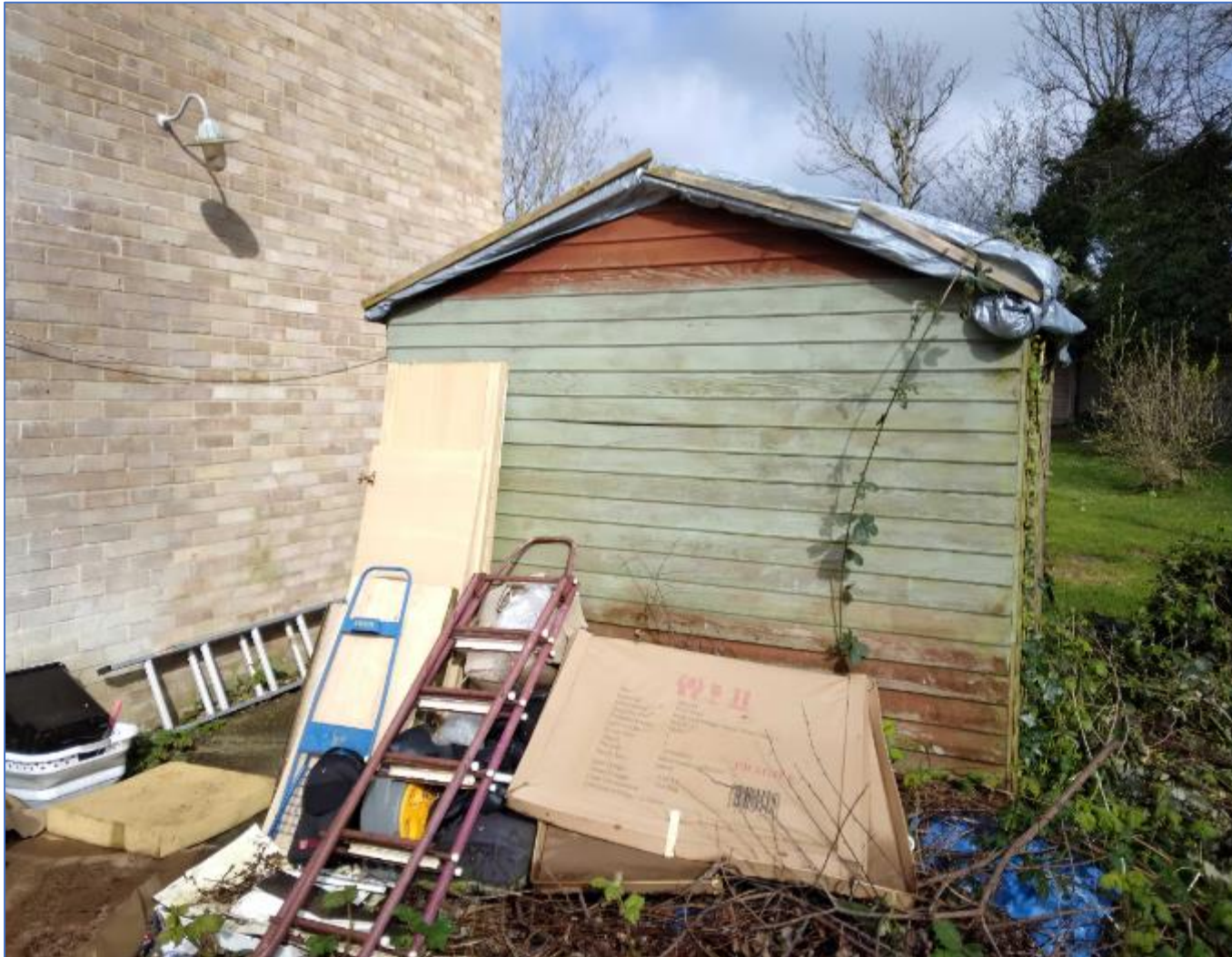
Photo 2: south facing elevation of the wooden shed.
