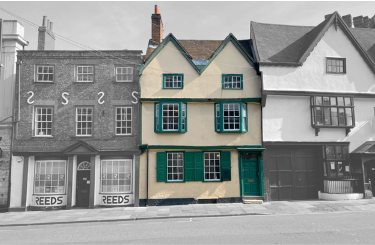
STREET FRONTAGE OF 15 CASTLE STREET
