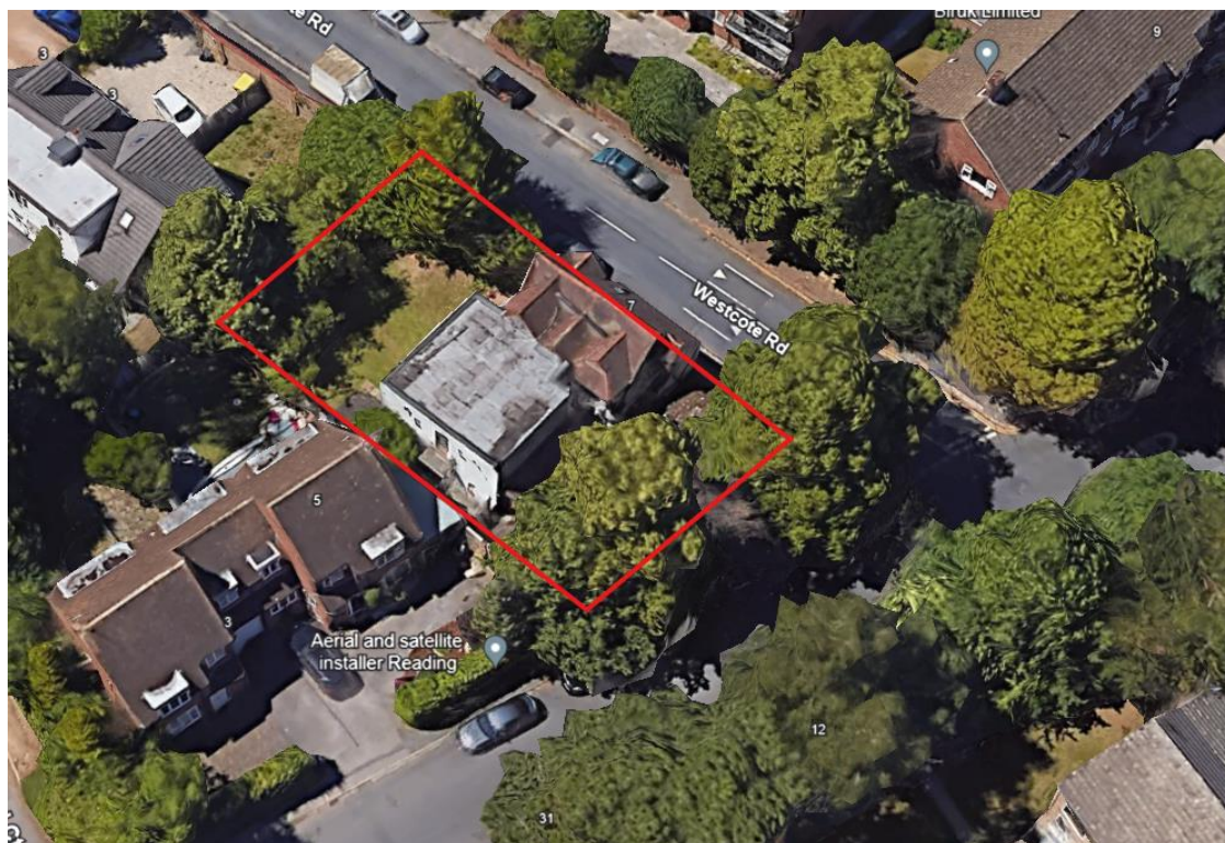
Application site, image taken from Google Earth on 17 June 2024.
