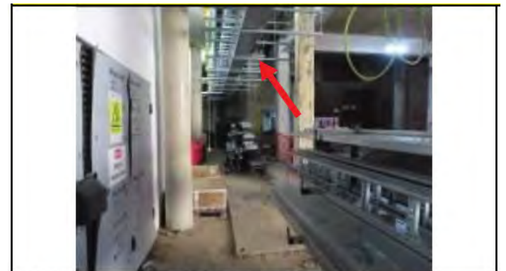
P2 Undercroft under slung services next to Thames Tower road access. Localised bird netting recommended.
