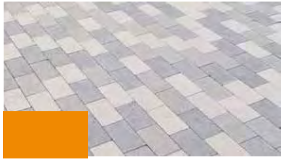
P9 - Block paving to Main Entrances; Size: 200x100x60mm, Colour: Light Grey and Mid Grey, Laying Pattern: Stretcher bond
