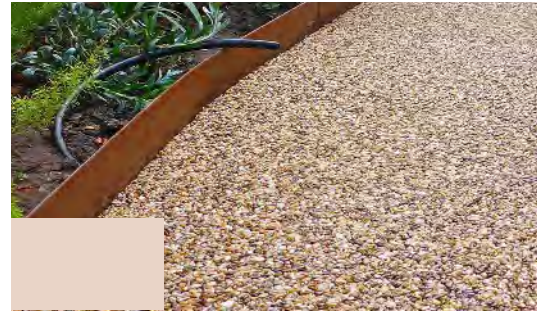
P8 - Pocket Park Pathway Resin bound gravel; Colour; Silver/Buff
