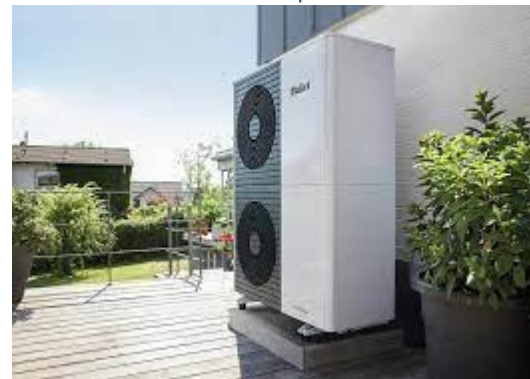
Figure 9: Air Source Heat Pump
