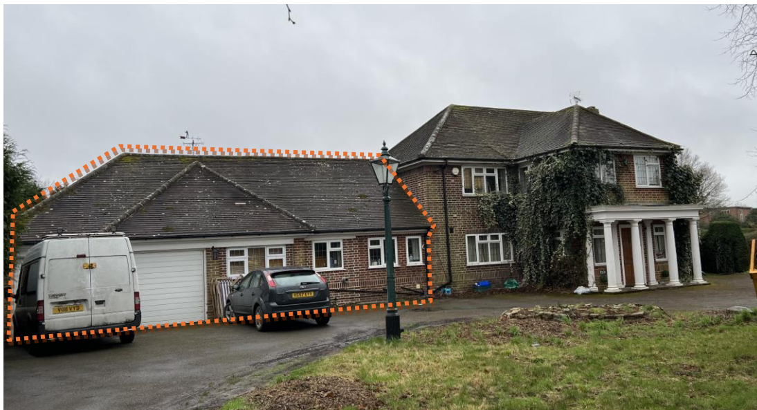
Figure 9 – Photograph of the existing dwelling, with the area to be demolished identified in orange dashed line.
