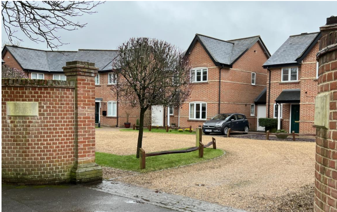
Figure 11 – Photograph of Bell Court development showing architectural details such as brick banding, brick headers and column detailing.
