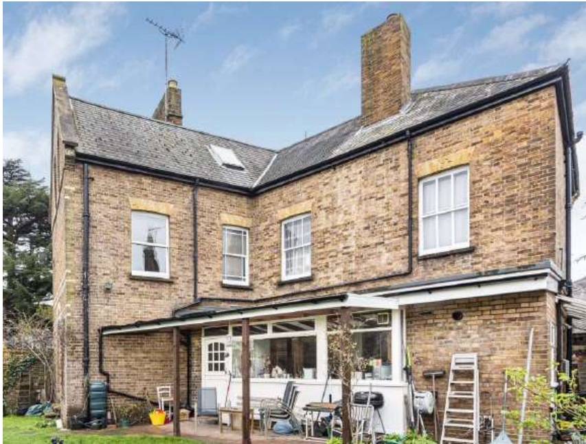
Photo Flat roof Extension over existing kitchen area
