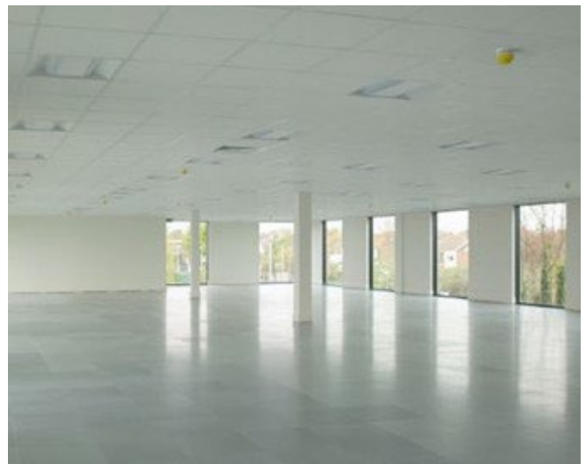
Indicative image of raised flooring
