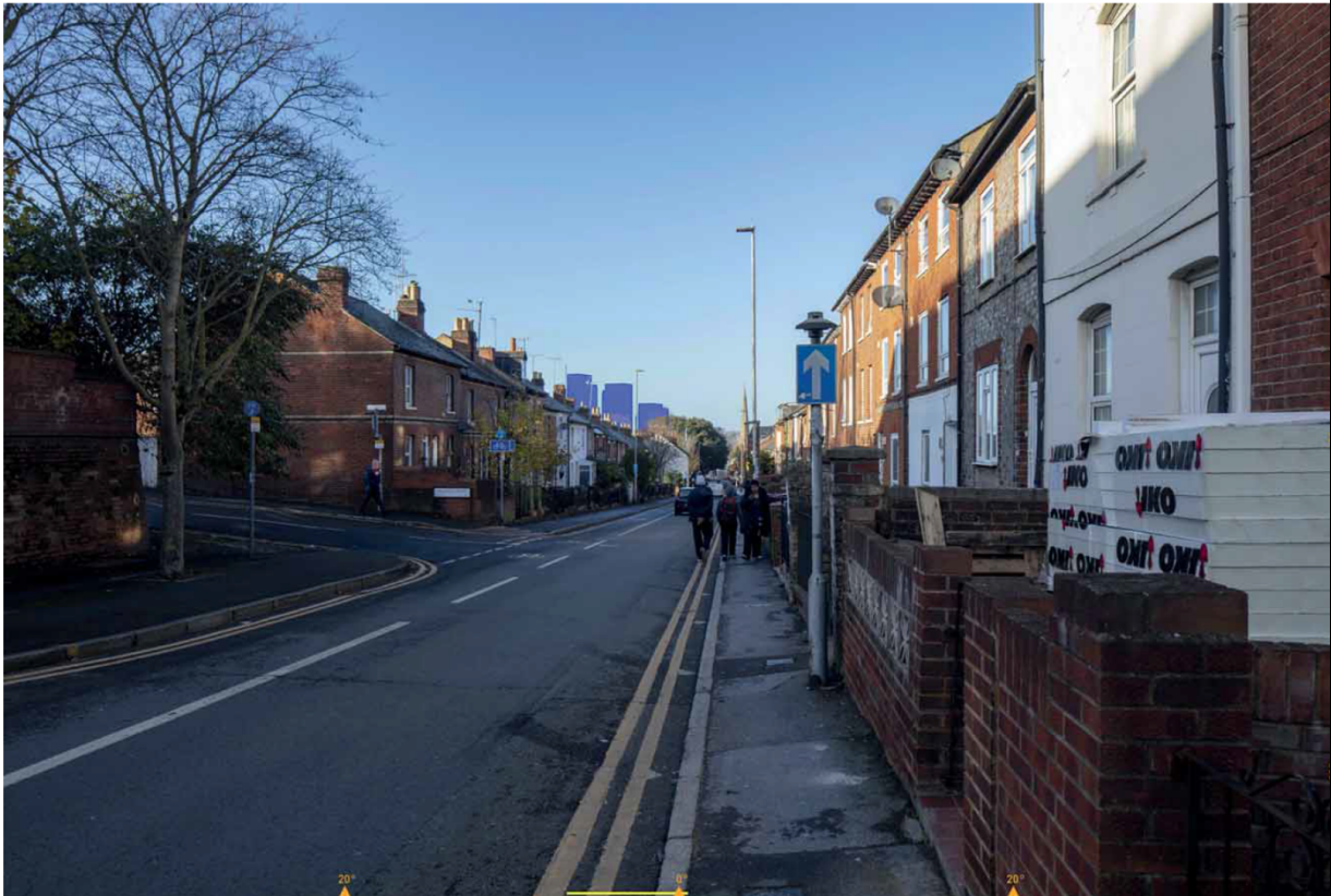
View from the top of Southampton Street post development. From EIA Volume 2
