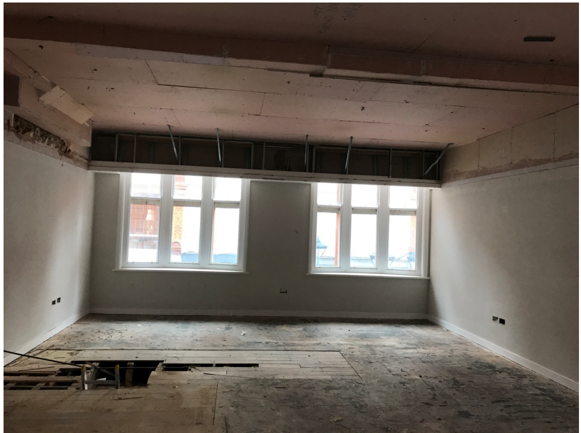
Typical Existing First, Second & Third Floors facing Queen Victoria Street:
