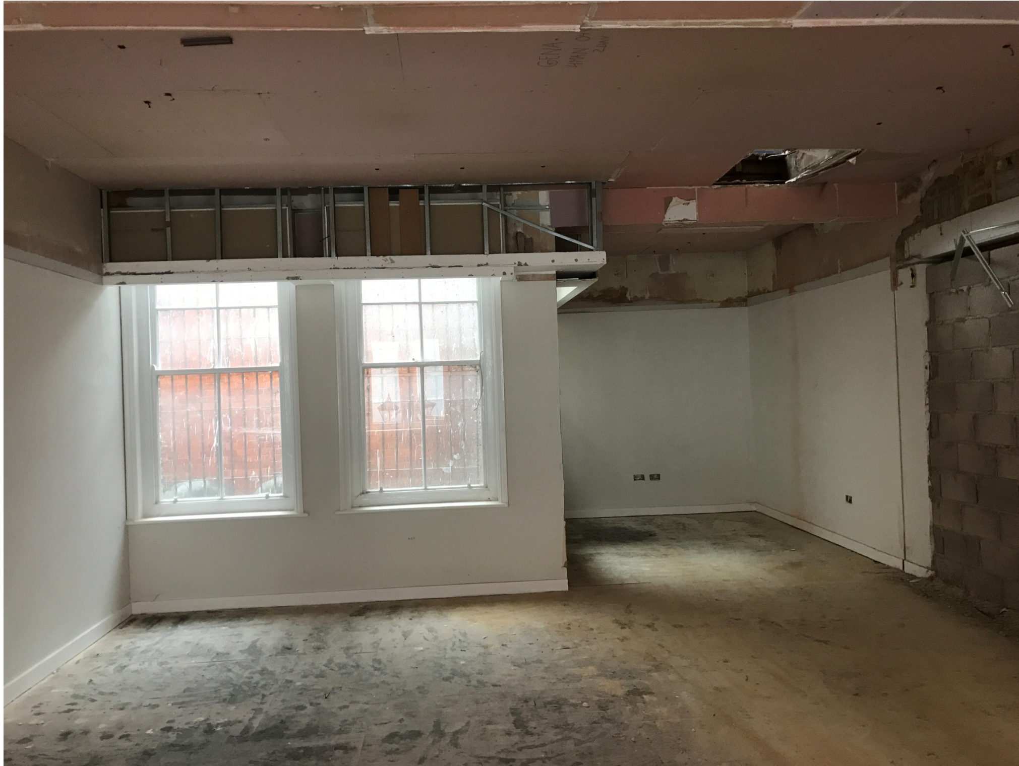
Typical First, Second & Third Floors – Looking East towards the light well:
