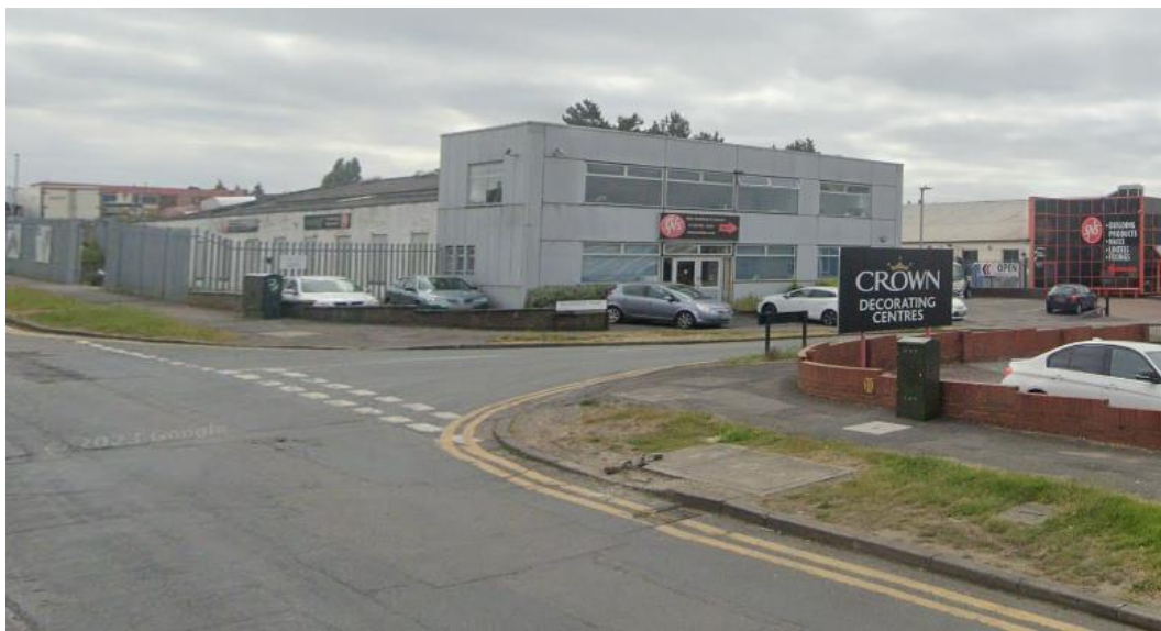
Existing site view.
