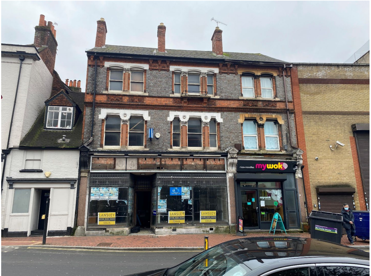
Existing Front Elevation – View from Friar Street
