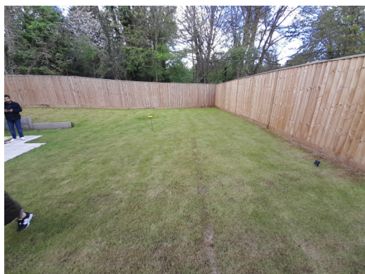
Looking north, decking will be located where fence lines meet.
