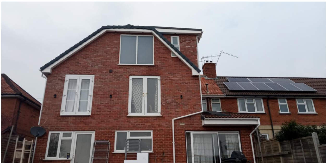
Photograph of completed works, taken by case officer on 07/03/2024
