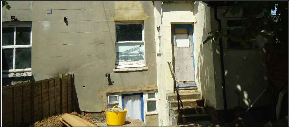
Photo of Rear Lower Ground Floor
