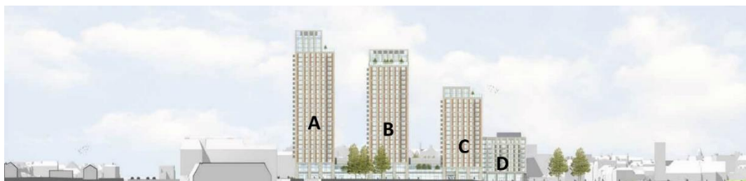
Figure 4: Building identification. Image from application.
