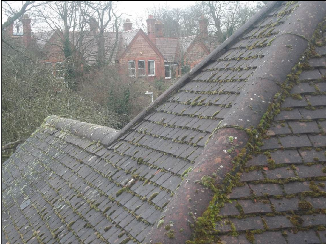
Figure 5. Example of ridge and hip tiles. 8 Avebury Square, Reading. 13.02.24
