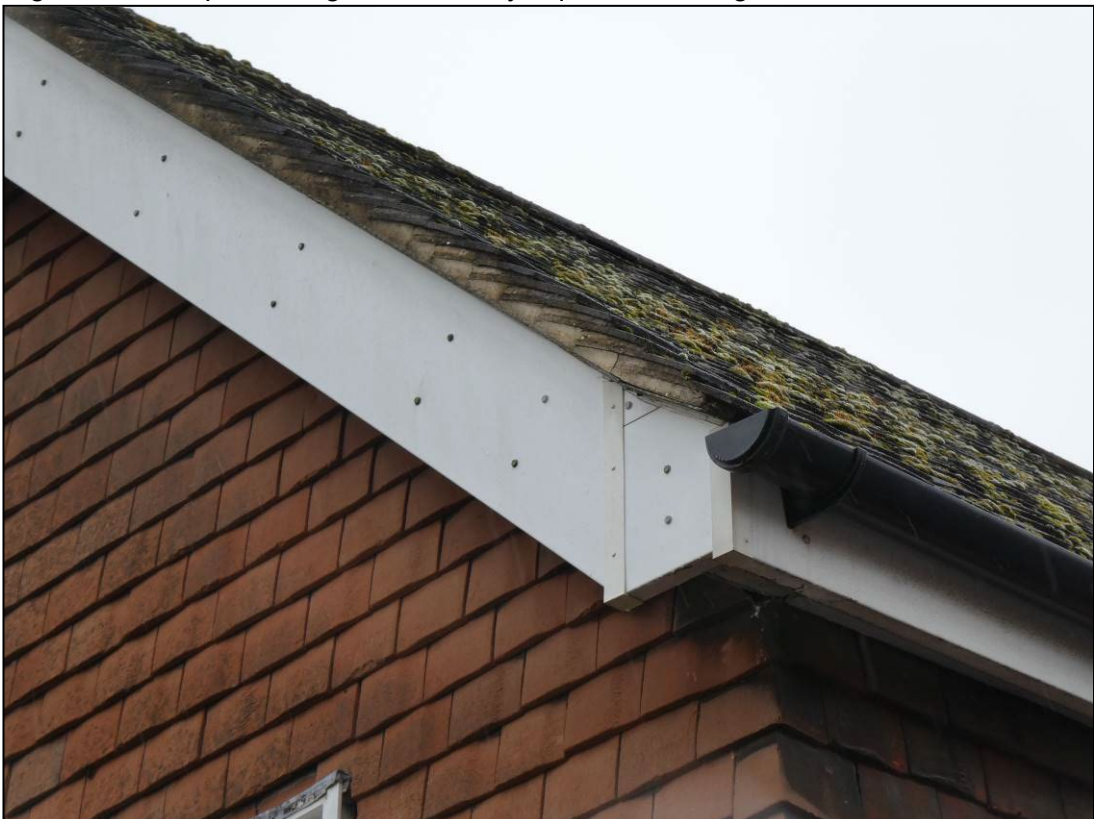
Figure 6. Example of verges. 8 Avebury Square, Reading. 13.02.24
