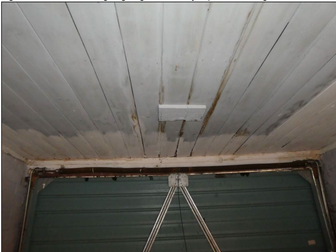
Figure 15. Boarded ceiling of garage. 8 Avebury Square, Reading. 13.02.24
