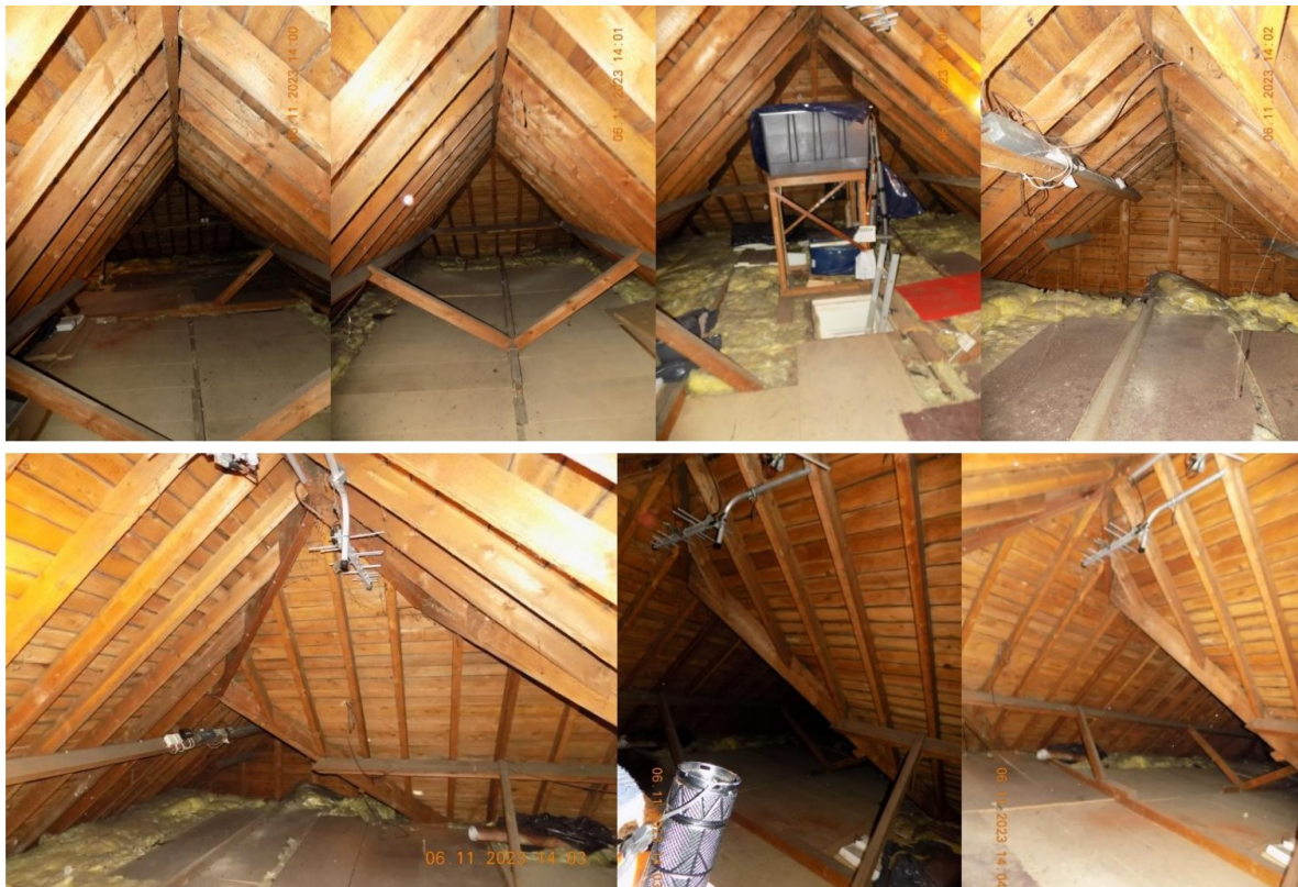
Image 8 – Internal views from within the main roof void spaces of the property
