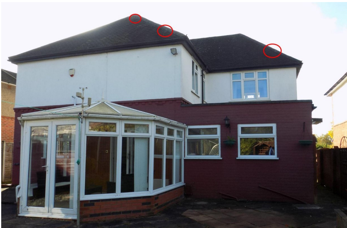
Image 4 – Rear North/East facing elevation of the property offering further gaps of value within the roof coverings
