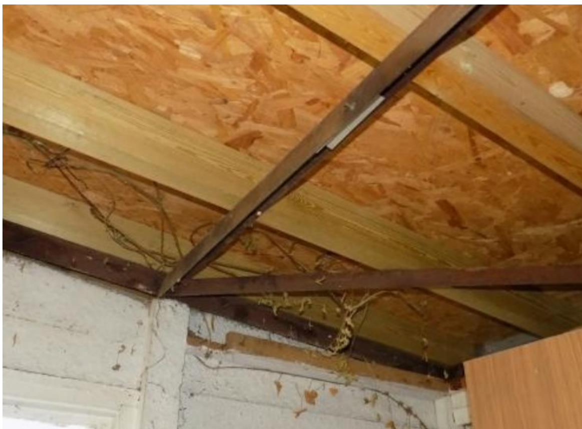
Image 9 – Internal view from within the rear garage outbuilding which offers a flat roof coverings
