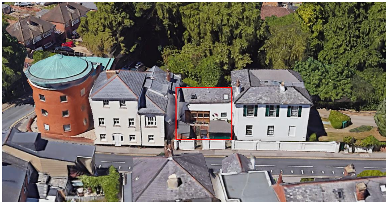
Flat 12 of 52 Tilehurst Road indicated in red, bounded by the main building of number 52 Tilehurst Road to the right, and number 54 Tilehurst Road to the left.
