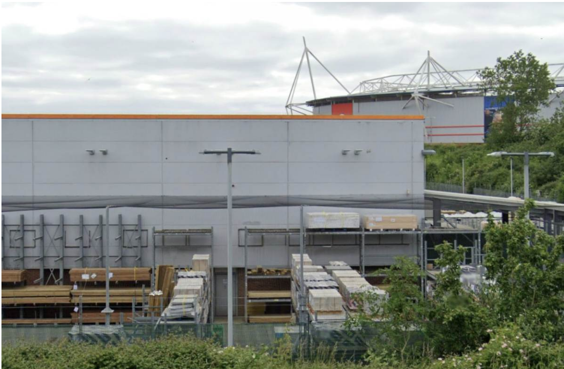
EXISTING REAR ELV
