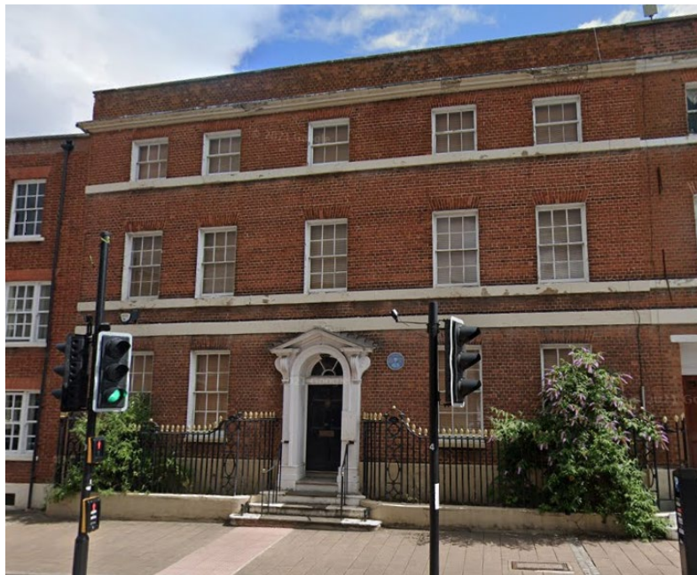
Photo 1 – View of the front elevation
