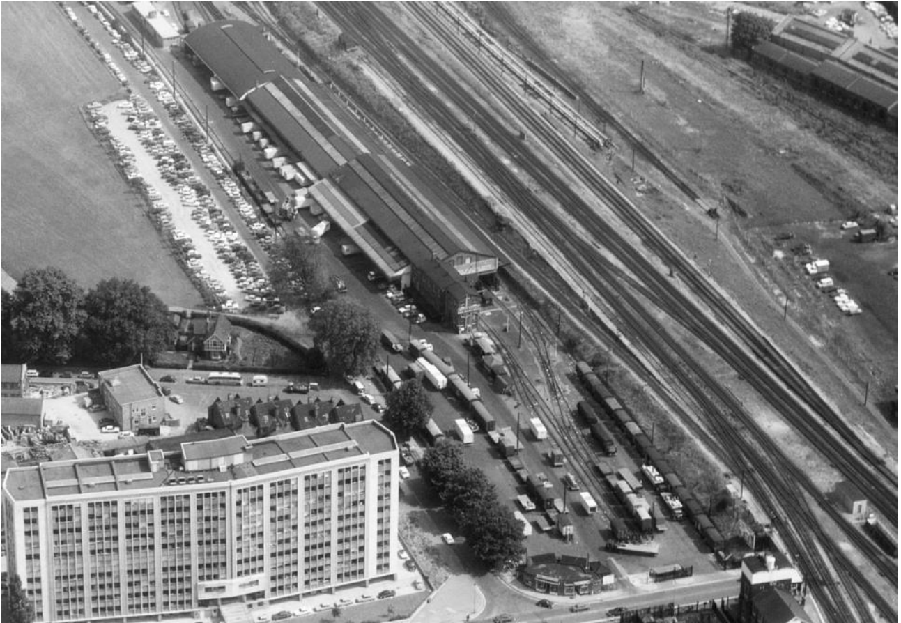
Figure 6 – Cars parked on the southern edge of King’s Meadow in 1962 (Aerofilms EAW098027, flown 13 March 1962). Reading Bridge House is in the foreground.
