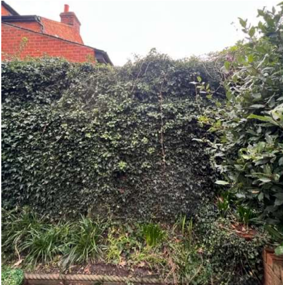
The height of garden wall can be seen in relation to it sitting above the new bifold doors in the extension at number 26 Priest Hill
