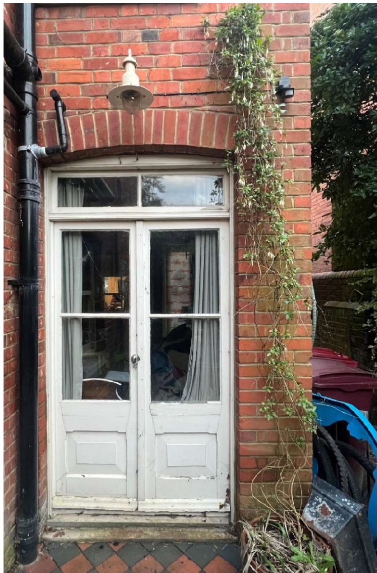
This original glazed garden door with raised and fielded panelling, glazed transom, brick arch and brick wall to the right, are all to be restored and made a feature within the new extension
