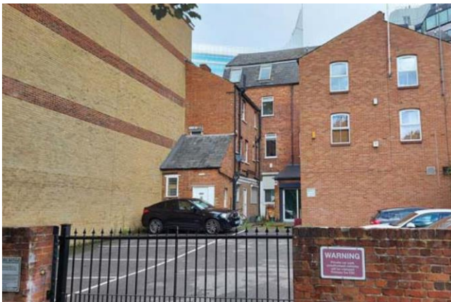
Figure 1 - View of the site
