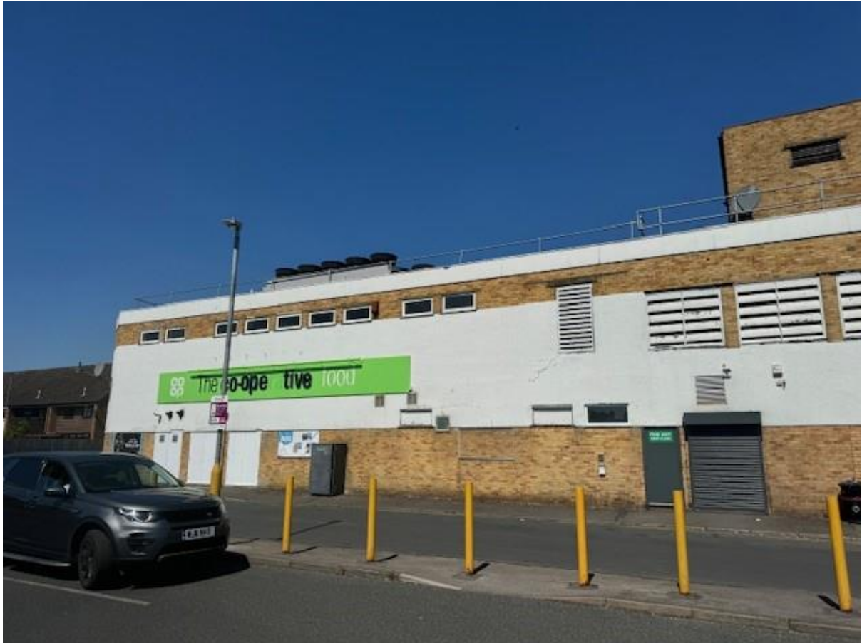
Site Visit Photos taken on 25 th of June 2024
