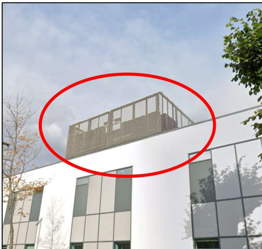
Figure 2 – View from Redlands Road
