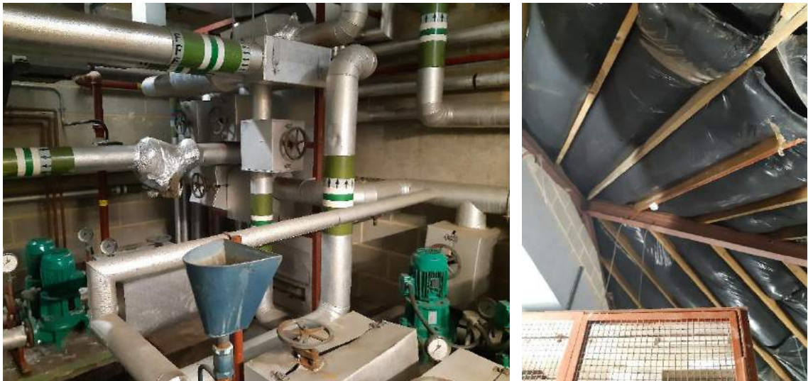
Image 6 (left): Middle section of roof voids. Image 7 (right): Insulation between support beams
