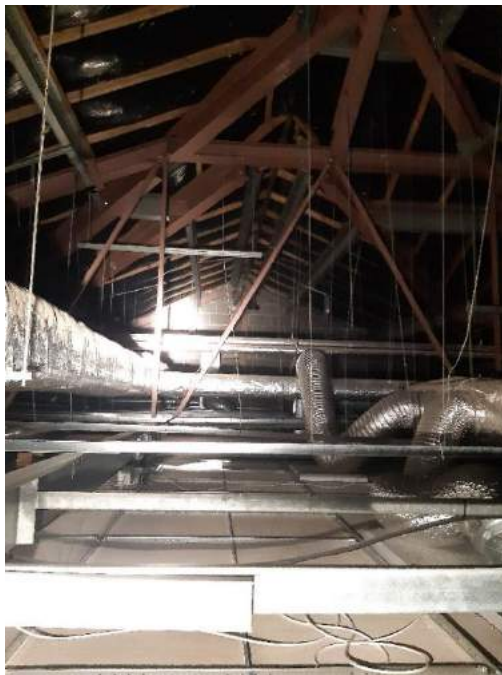
Image 10: Internal environment within the west and east sections of the roof voids.
