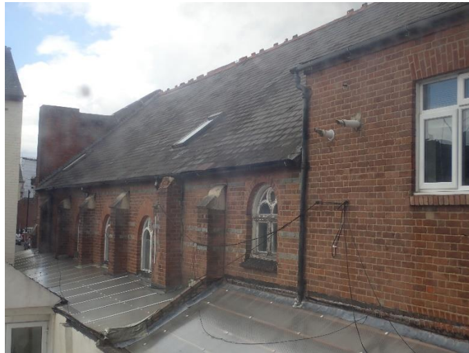
Photo 1: Showing pitched tiled roof
