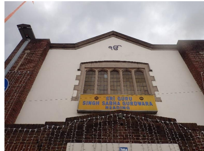
Photo 2: Showing front façade of the building.
