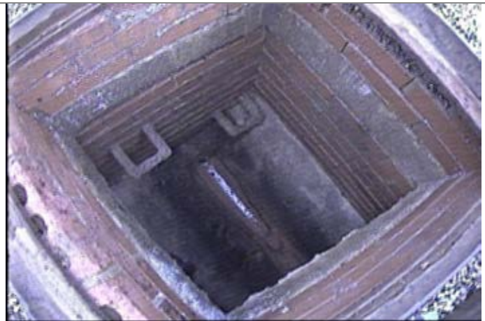
Manhole / Access Point: FWMH1A Internal
