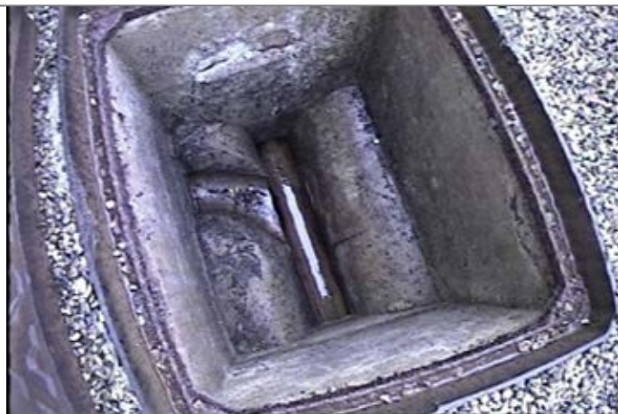
Manhole / Access Point: FWMH1 Internal
