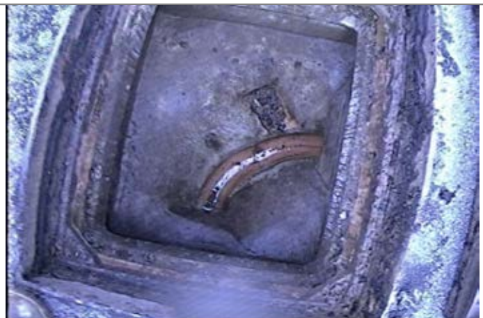
Manhole / Access Point: FWMH12 Internal
