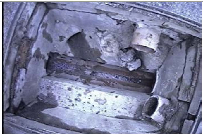
Manhole / Access Point: SWMH10 Internal
