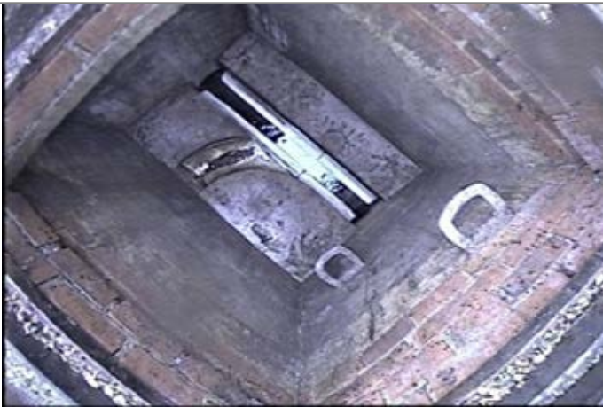
Manhole / Access Point: FWMH5 Internal
