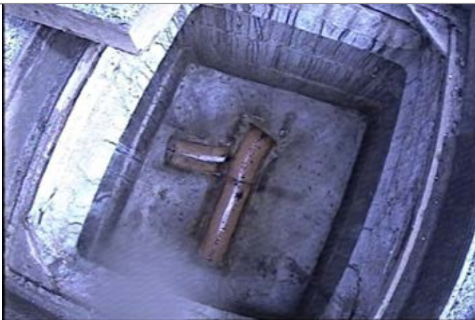
Manhole / Access Point: FWMH11 Internal
