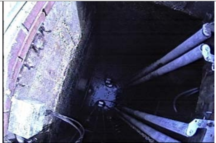
Manhole / Access Point: PUMP STATION Internal
