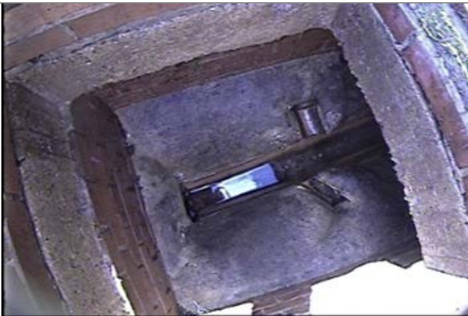
Manhole / Access Point: FWMH1B Internal
