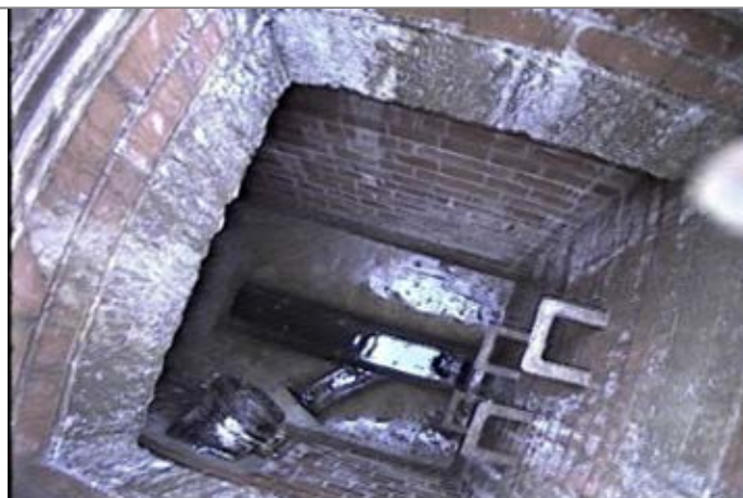
Manhole / Access Point: SWMH4 Internal
