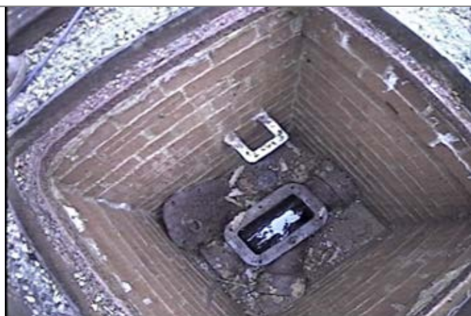
Manhole / Access Point: FWMH3 Internal
