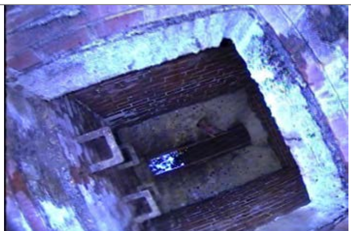
Manhole / Access Point: SWMH14 Internal
