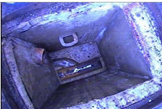
Manhole / Access Point: SWMH12 Internal
