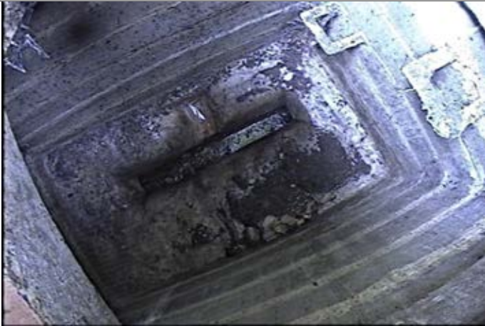
Manhole / Access Point: FWMH9 Internal
