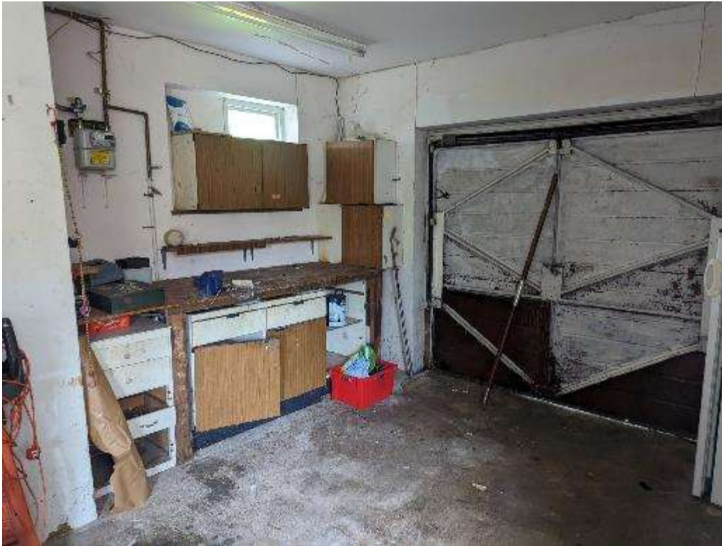
View of Garage
