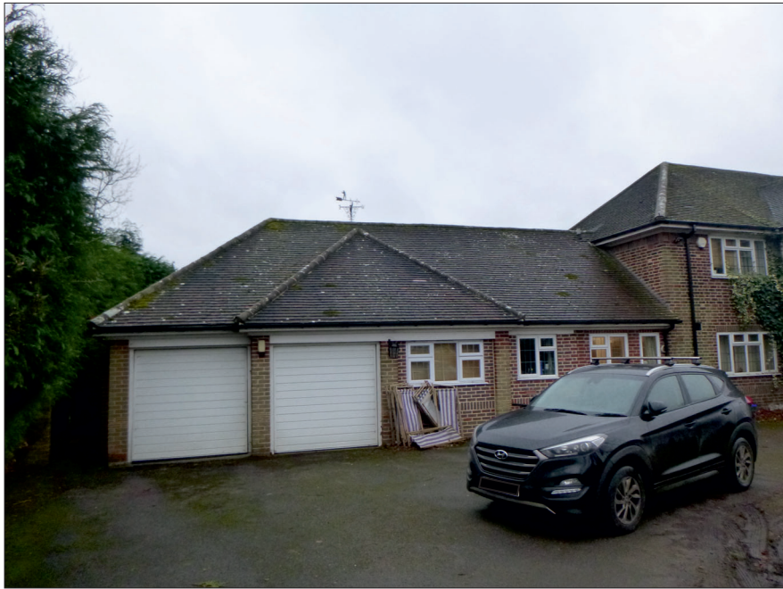
Photograph 2: Showing the front of the attached Annexe/Garages (B2).
