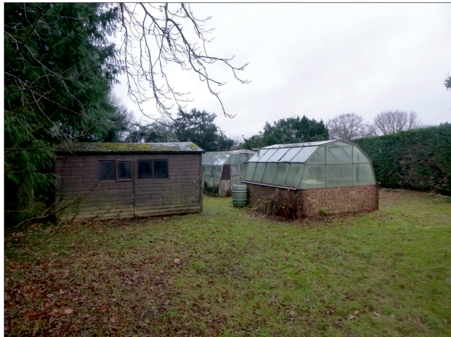
Photograph 7: Showing a number of outbuildings (B4, 5 & 6) set within the garden area.
