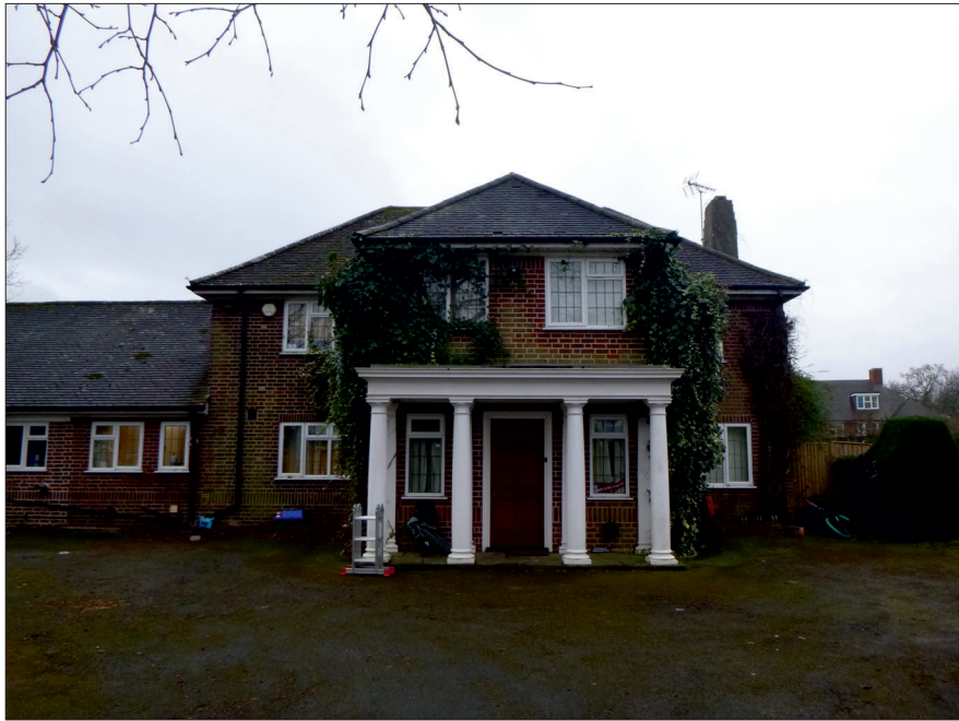
Photograph 1: Showing the front of the Residential Dwelling (B1).
