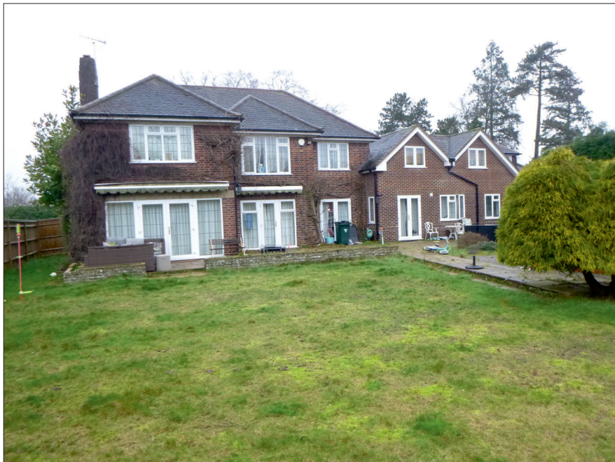
Photograph 3: Showing the rear of the Residential Dwelling (B1) and attached Annexe/ Garages (B2), with well-maintained garden.
