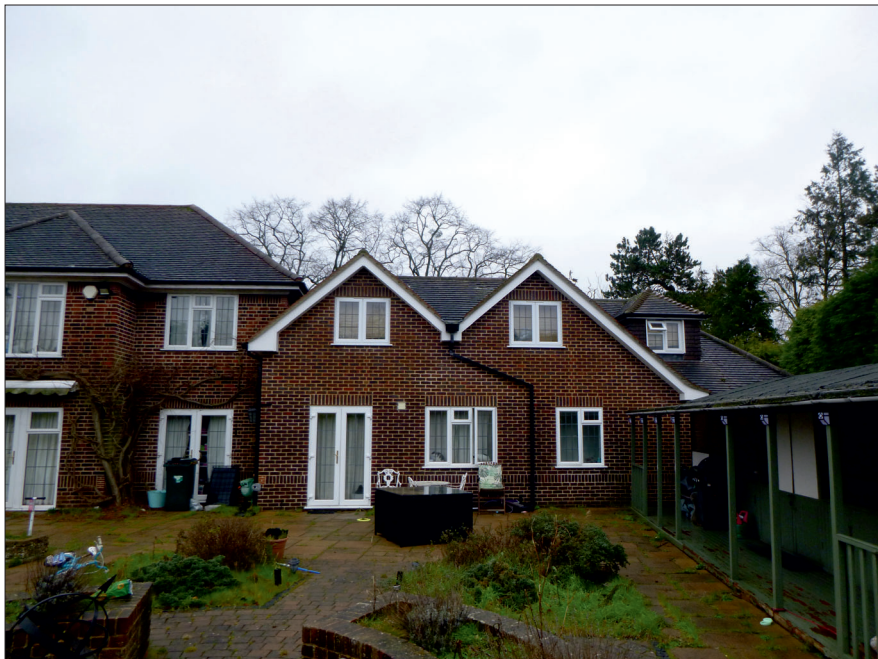
Photograph 4: Showing the rear of the Annexe/Garages (B2), with well-sealed cheek tile hanging and adjacent outbuilding (B3).
