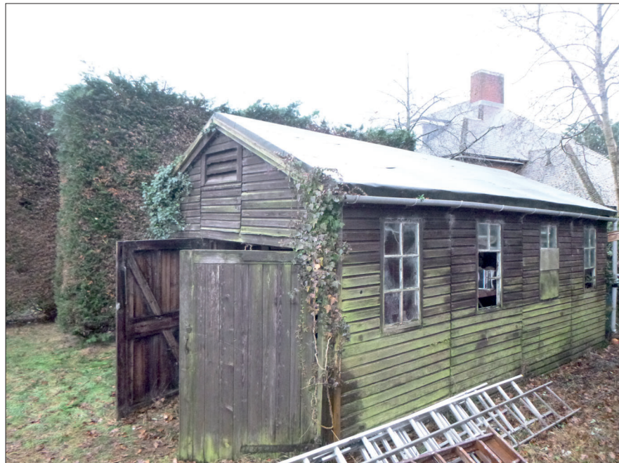
Photograph 8: Showing the timber constructed store (B9).
