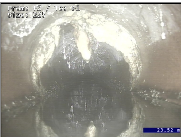
Attached deposits, encrustation from 9 to 3 o'clock 25% cross-sectional area loss
