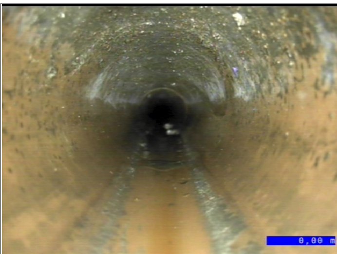
Water level 0% height/diameter
