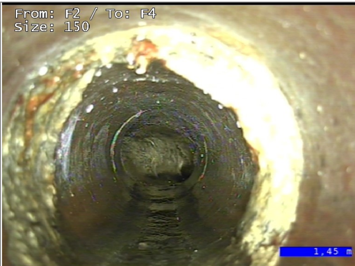
Attached deposits, encrustation from 11 to 5 o'clock 10% cross-sectional area loss
