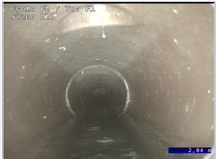
Junction at 12 o'clock, diameter 150mm
