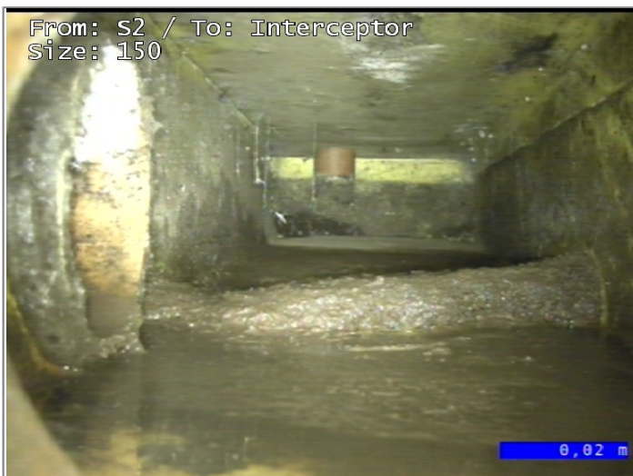
Finish node type, oil separator, reference Interceptor
