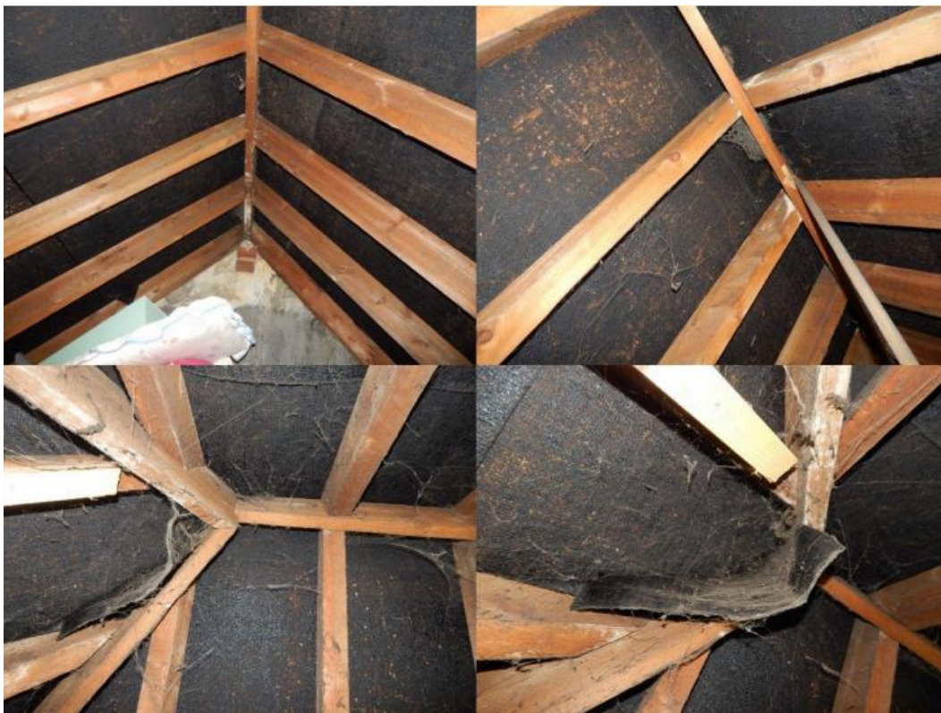
Image 10 – Internal view from within the main roof void spaces of the property
