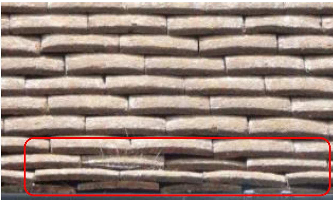
Image 2 – East facing elevation of the property which has demonstrated roof coverings which offer gaps of adequate proportions to offer likely shelter/access opportunities for bats throughout
