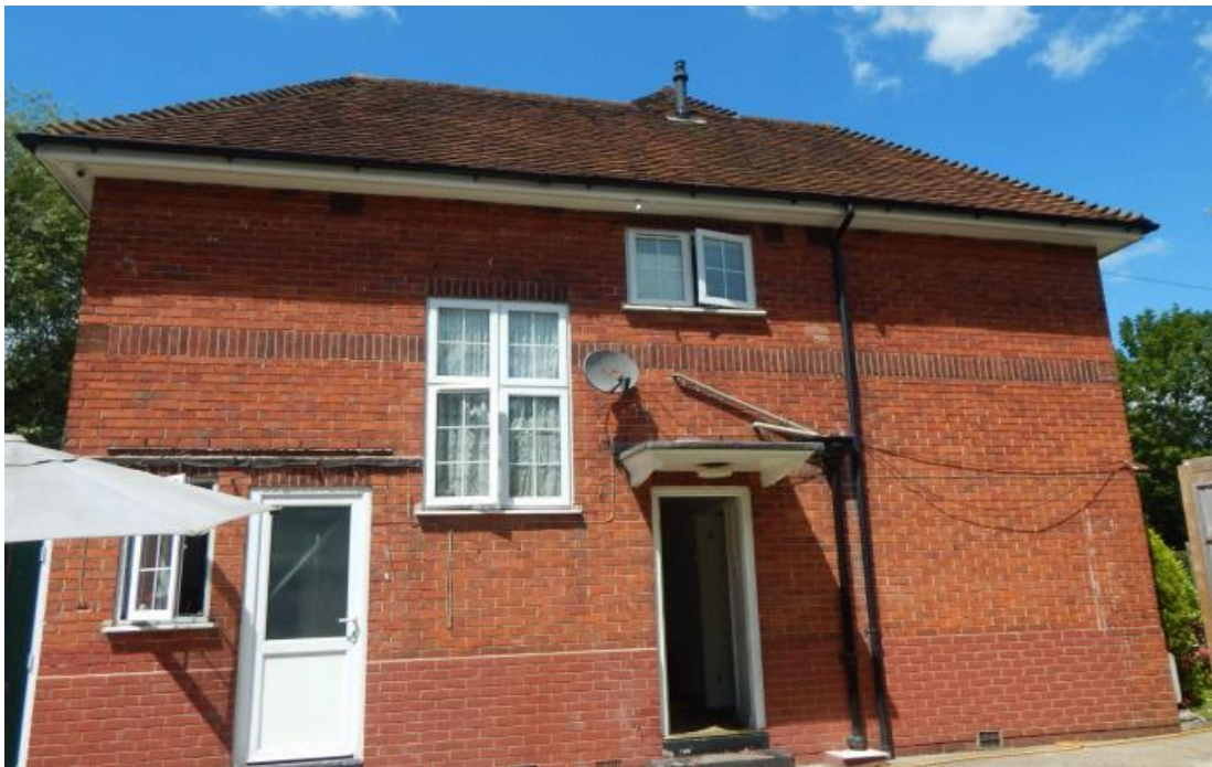
Image 6 – South facing elevation of the property
