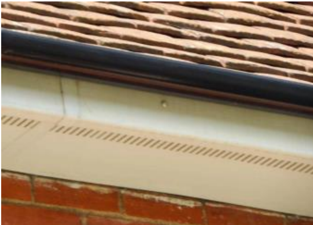
Image 8 – View of the eaves coverings which have demonstrated a fair condition throughout
