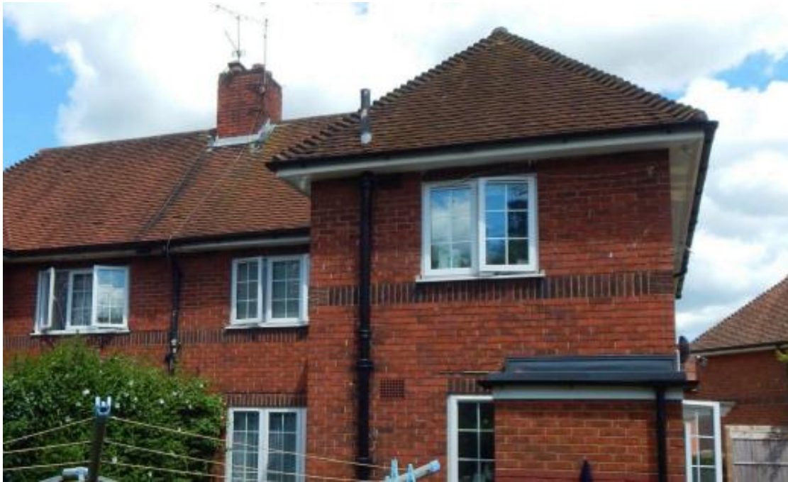
Image 3 – West facing elevation of the property
