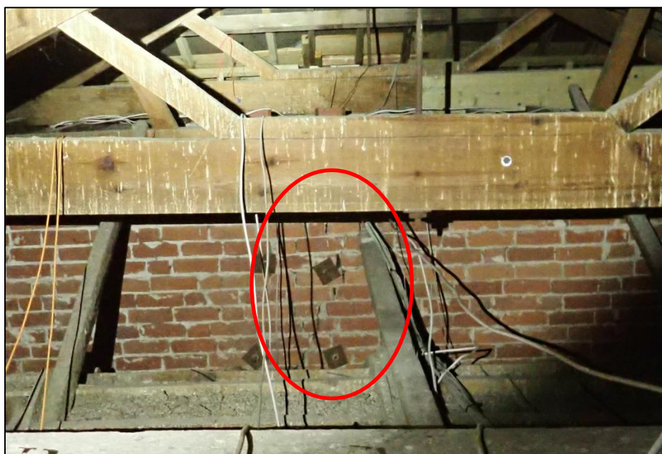
Figure 42. Cracking on the north wall of the archway.
