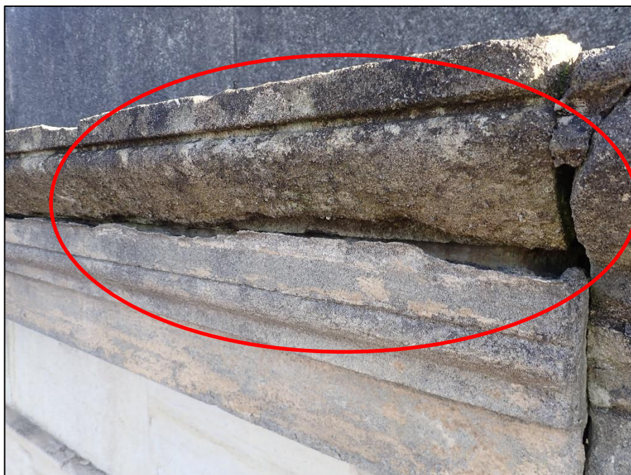
Figure 10. Partially detached section of repair (over the south lodge).
