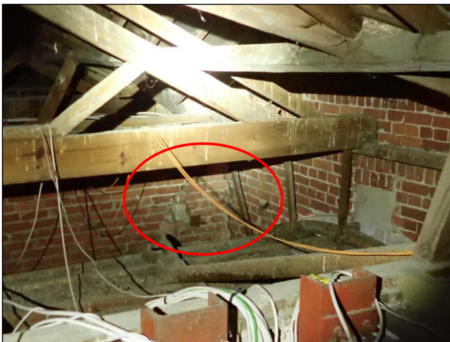
Figure 41. Cracking and dis-engagement of the brickwork in the south-west corner of the archway.
