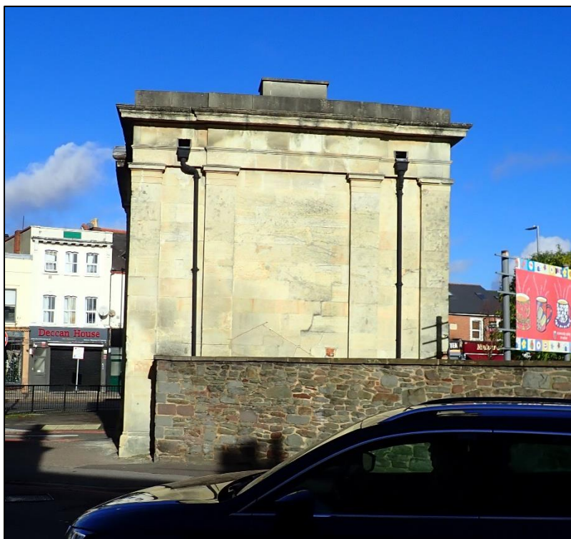
Figure 29. General view of the south elevation.
