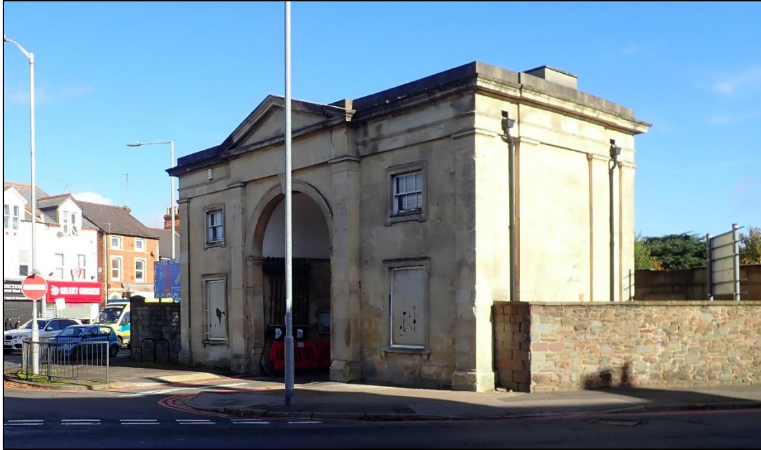
Figure 4. General view from the south-west.
