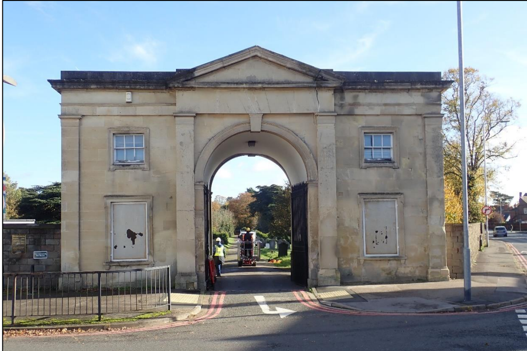
Figure 5. General view of the west elevation.
