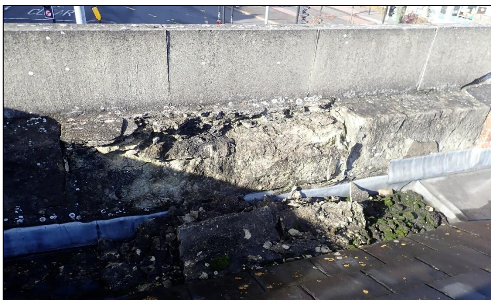
Figure 33. Fragmentation of the render and stone on the west
