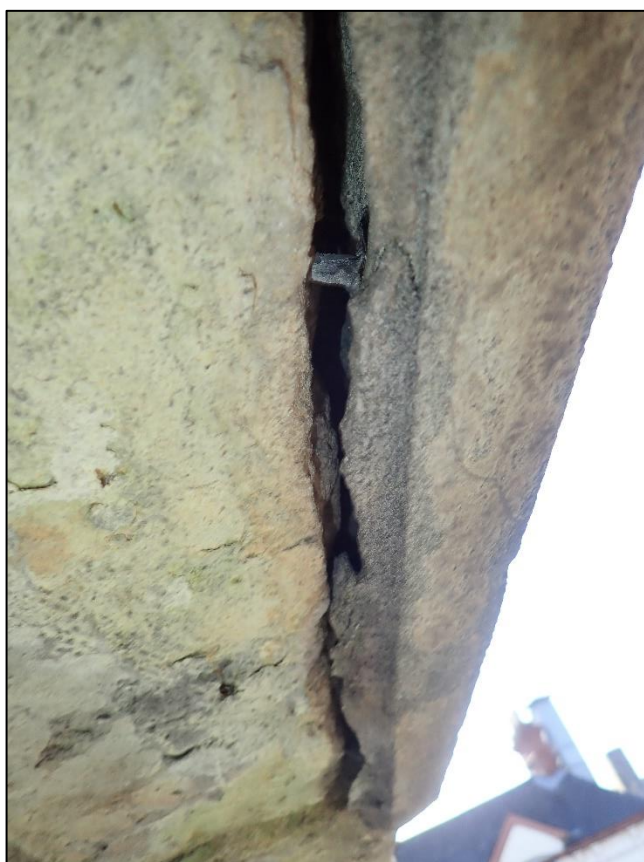
Figure 10. Partially detached section of repair (over the south lodge).
