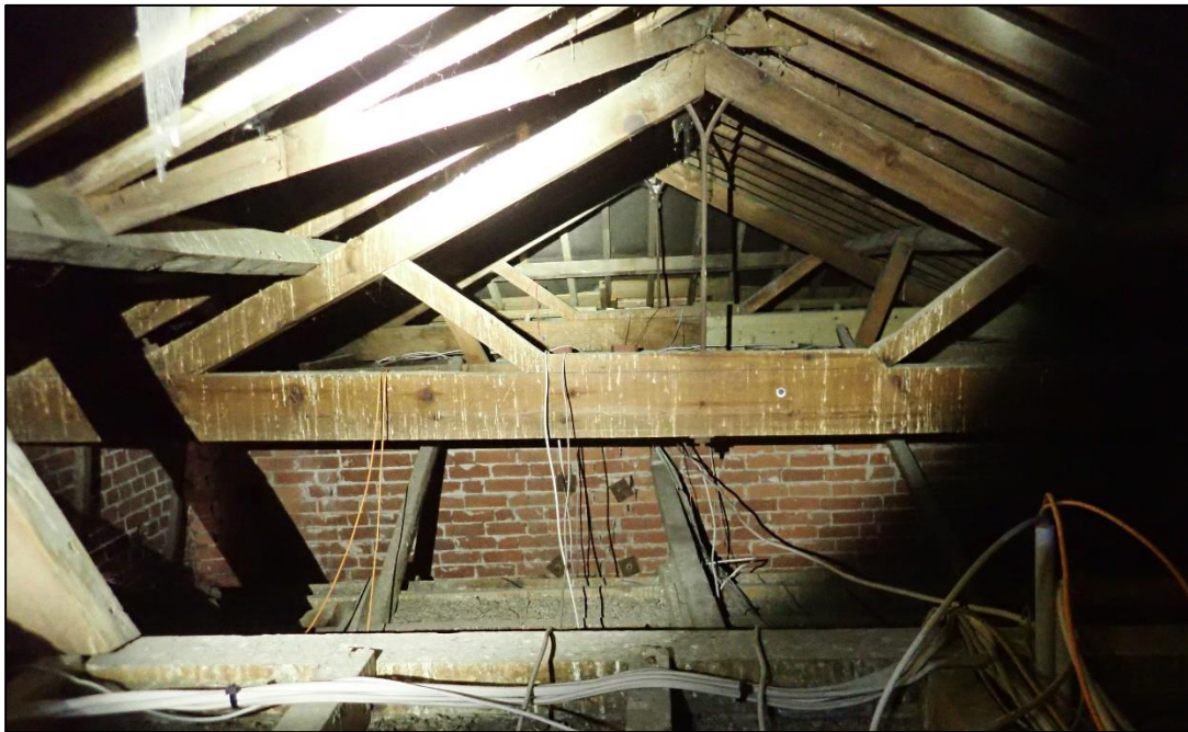
Figure 40. General view of the roof structure (Looking south from the northern access hatch).
