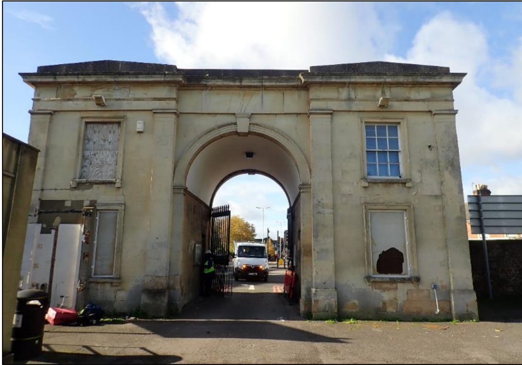
Figure 20. General view of the east elevation.
