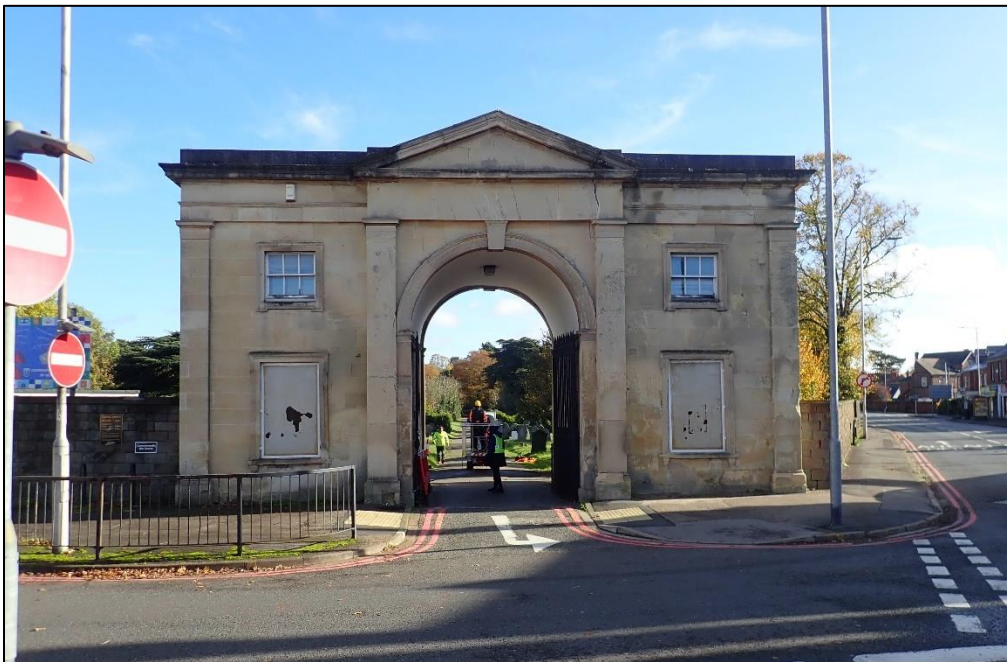
Figure 1. Principal (west) elevation of the Entrances Lodges at Reading Old Cemetery.
