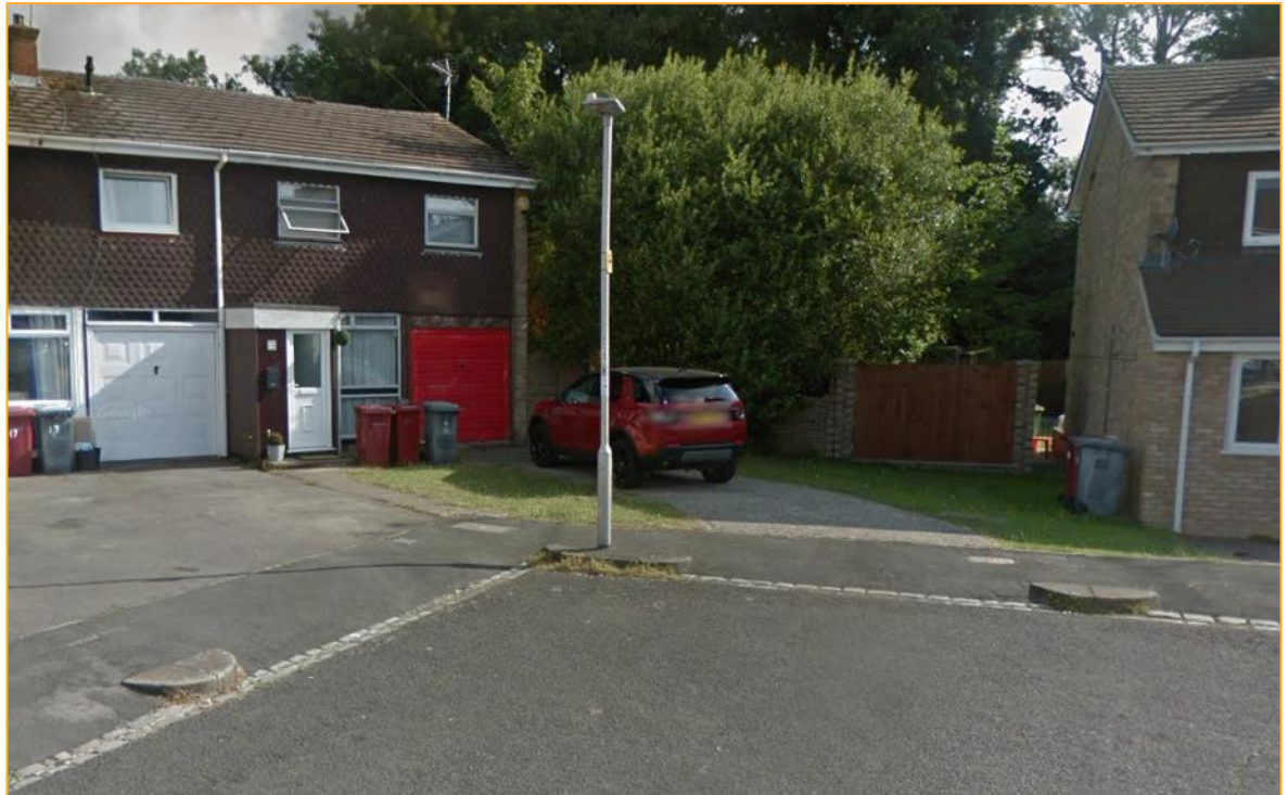
Figure 4.1 – Location of Existing Lamp Column.
