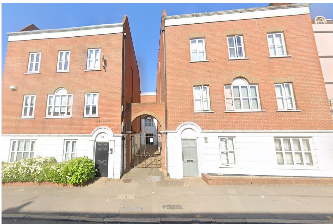
The application site as seen from Southampton Street. No. 87 Southampton Street is accessed by a footpath between nos. 85 and 89 Southampton Street.
