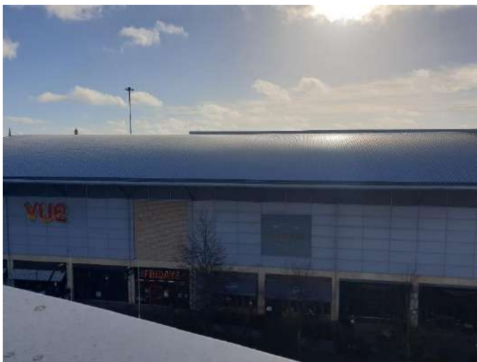
Photo 2: Northern elevation of B1.
