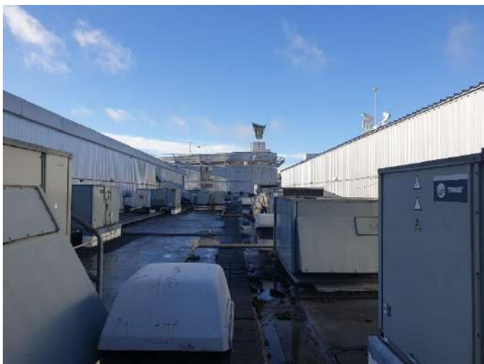
Photo 3: Roof of B1.
