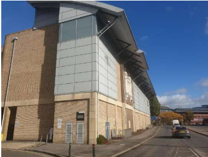
Photo 1: Southern and western elevations of B1.
