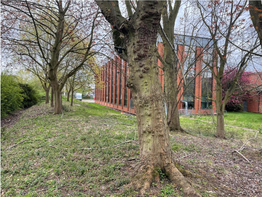
Photograph taken April 2023 showing dry ditch on left hand side.
