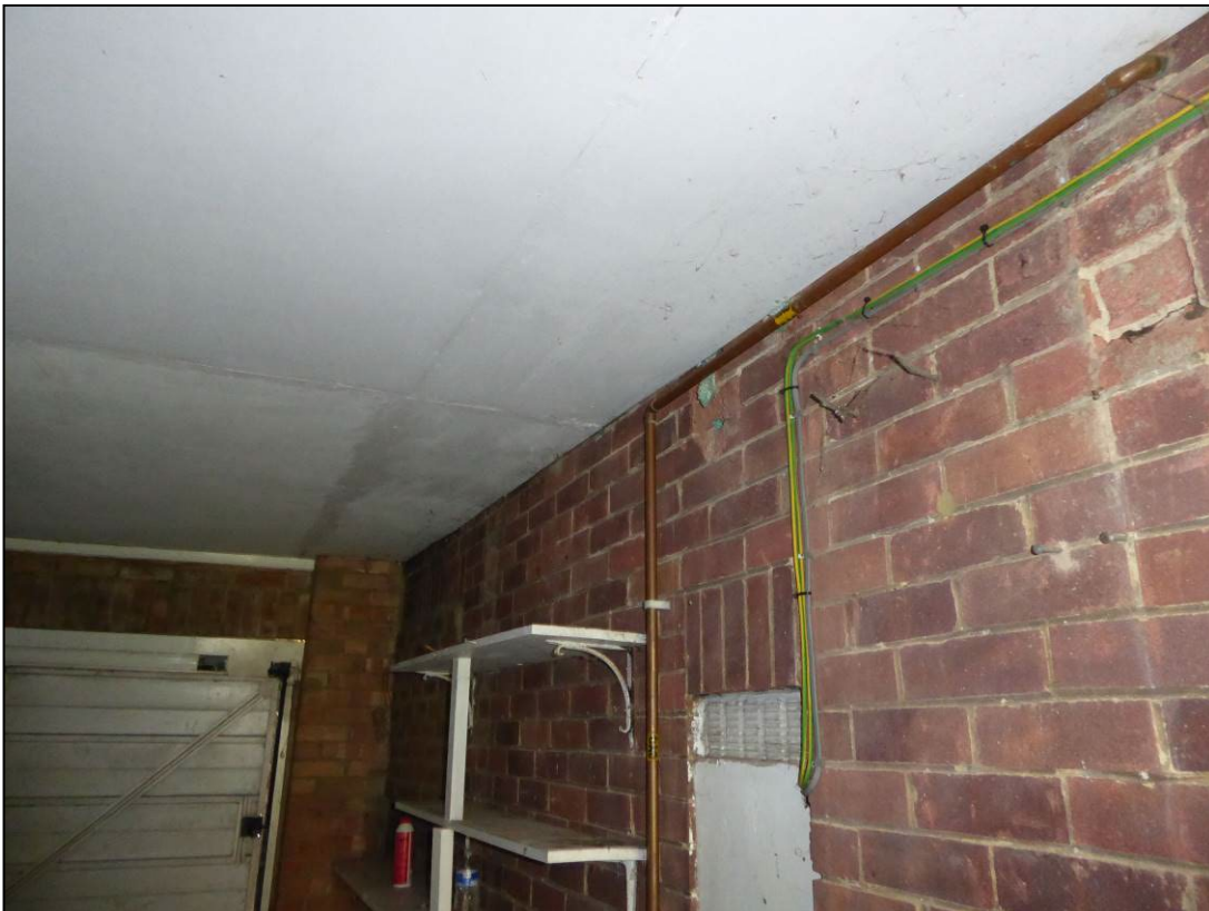
Figure 14. Boarded ceiling of garage roof. 48 Knights Way, Emmer Green. 07.05.24
