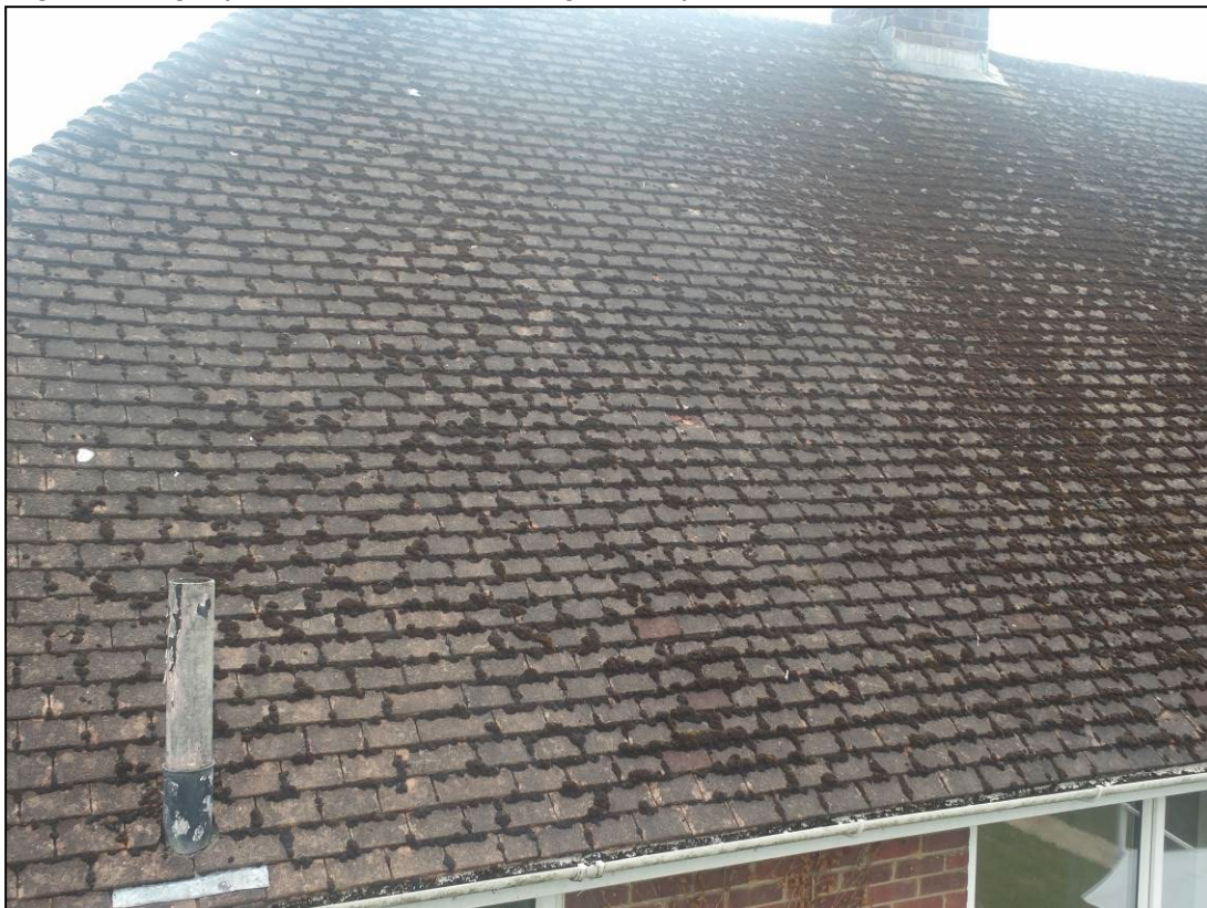
Figure 4. Tightly fitted roof tiles. 48 Knights Way, Emmer Green. 07.05.24
