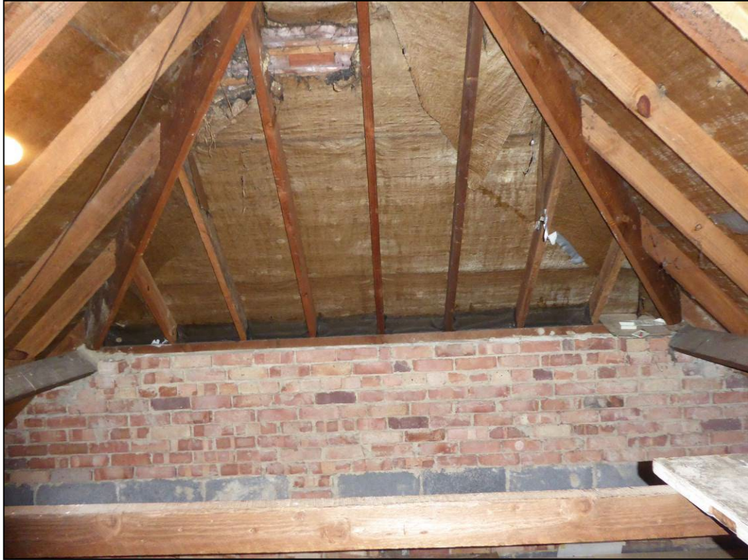
Figure 12. Example of ripped bitumen lining. 48 Knights Way, Emmer Green. 07.05.24
