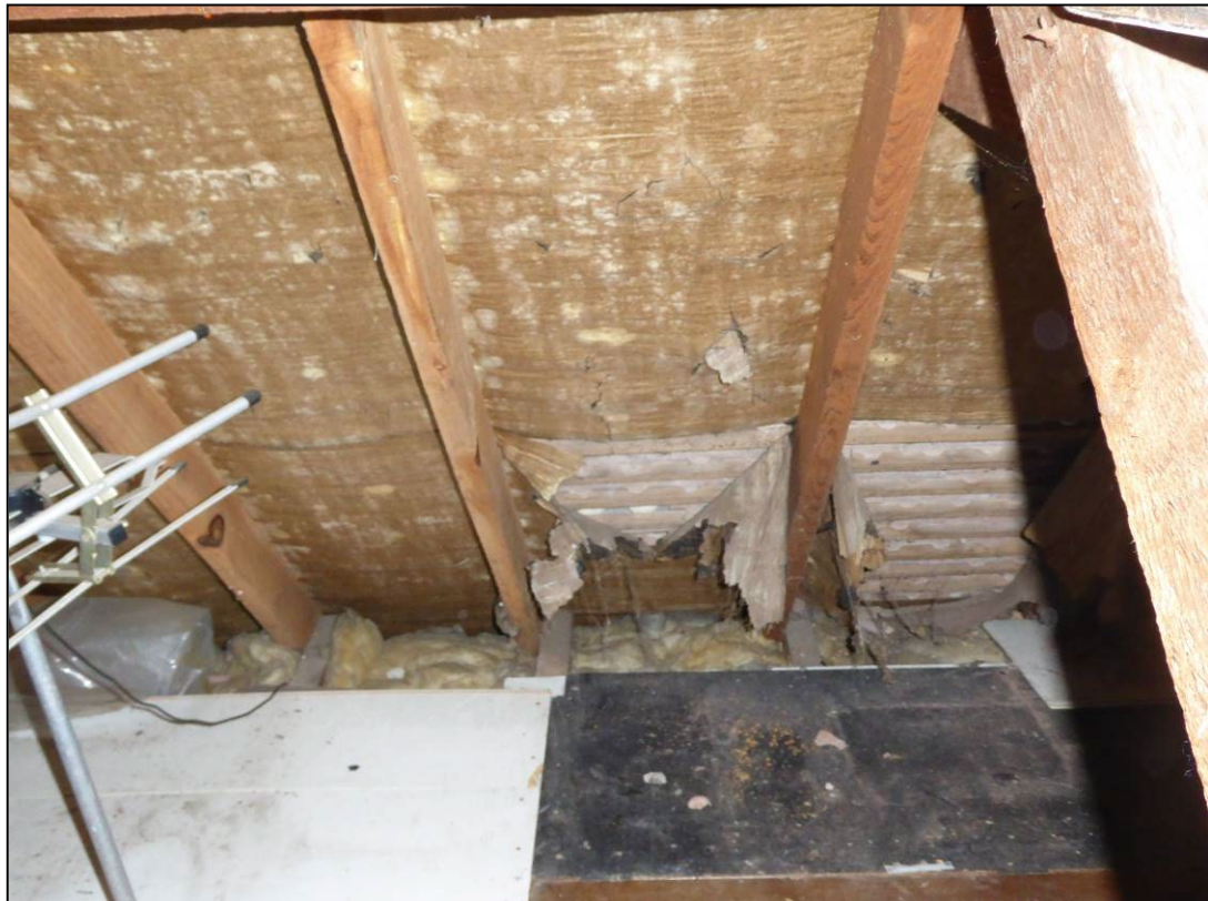
Figure 12. Example of ripped bitumen lining. 48 Knights Way, Emmer Green. 07.05.24
