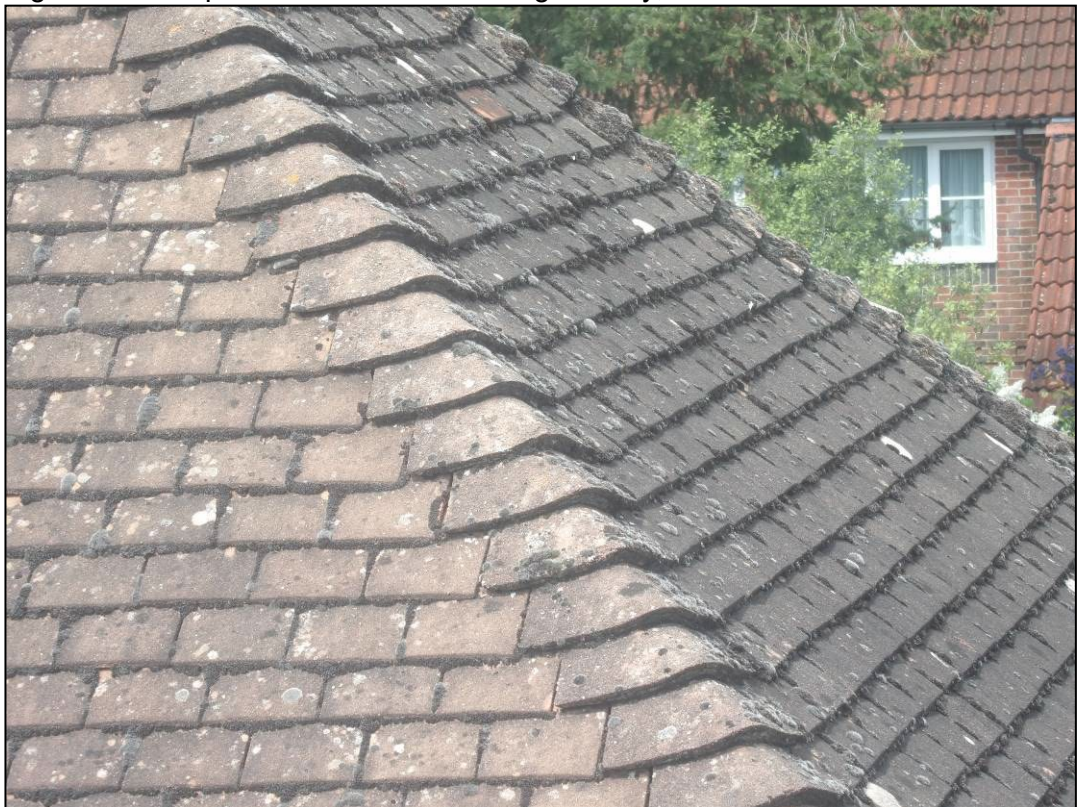
Figure 6. Example of bonnet tiles. 48 Knights Way, Emmer Green. 07.05.24
