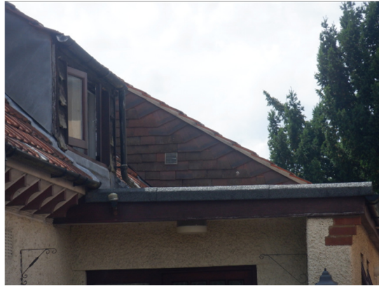
14. Bitumen felt flat roof sealed to timber fascia, viewed from the east.
