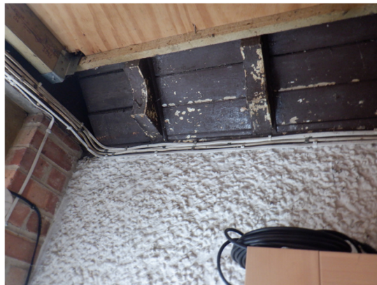
22. Timber soffit sealed to the internal rendered wall.
