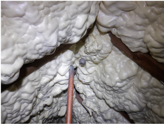
17. Lightly cobwebbed ridge heavily insulated with expanding foam.
