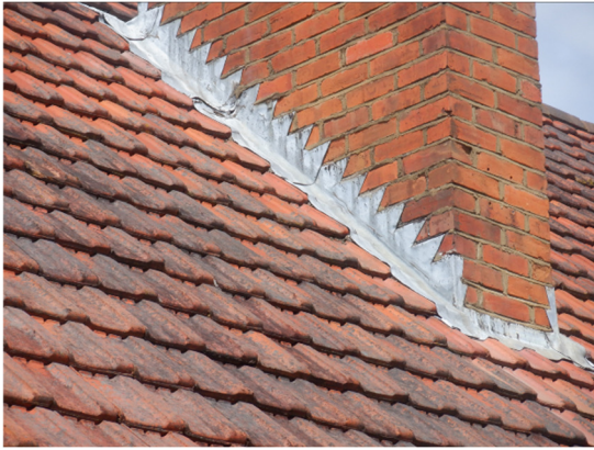
7. Lead flashing tight to the brickwork chimney and roof tiles, viewed from the southwest.
