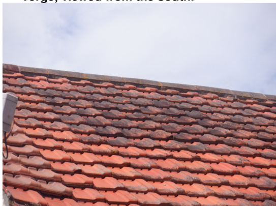
5. Fully intact ridge tiles, viewed from the southwest.
