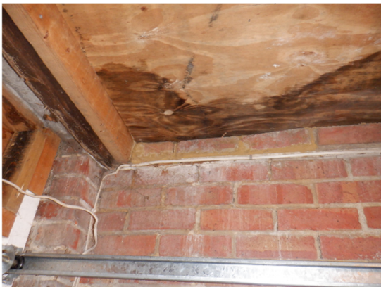
21. Garage lined with timber boarding that's sealed to the brickwork.
