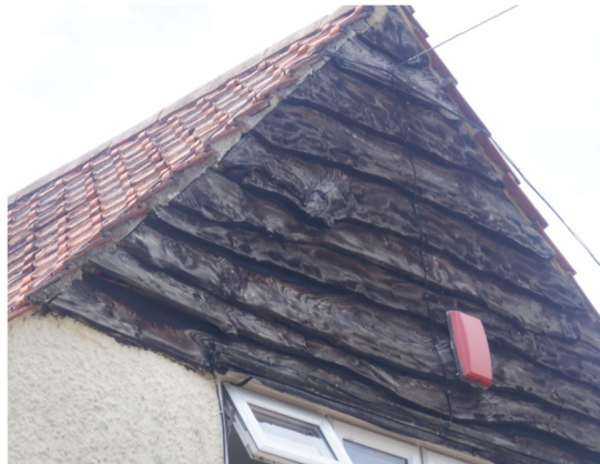
10. Lifted waney edge timbers on the front gable, viewed from the east.
