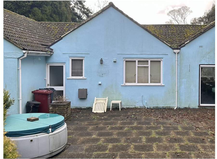
Figure 2: Existing rear elevation.
